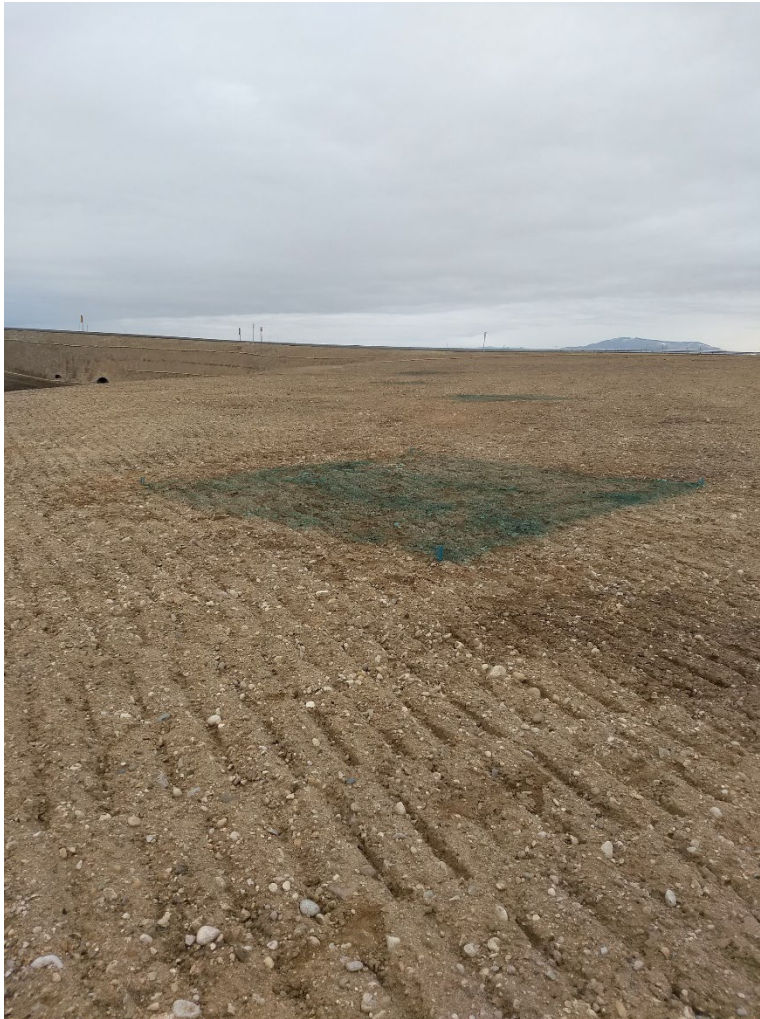
Figure 4.5 Battalion Pro® applied to I-84 Black's Creek area slated for hydroseeding.
