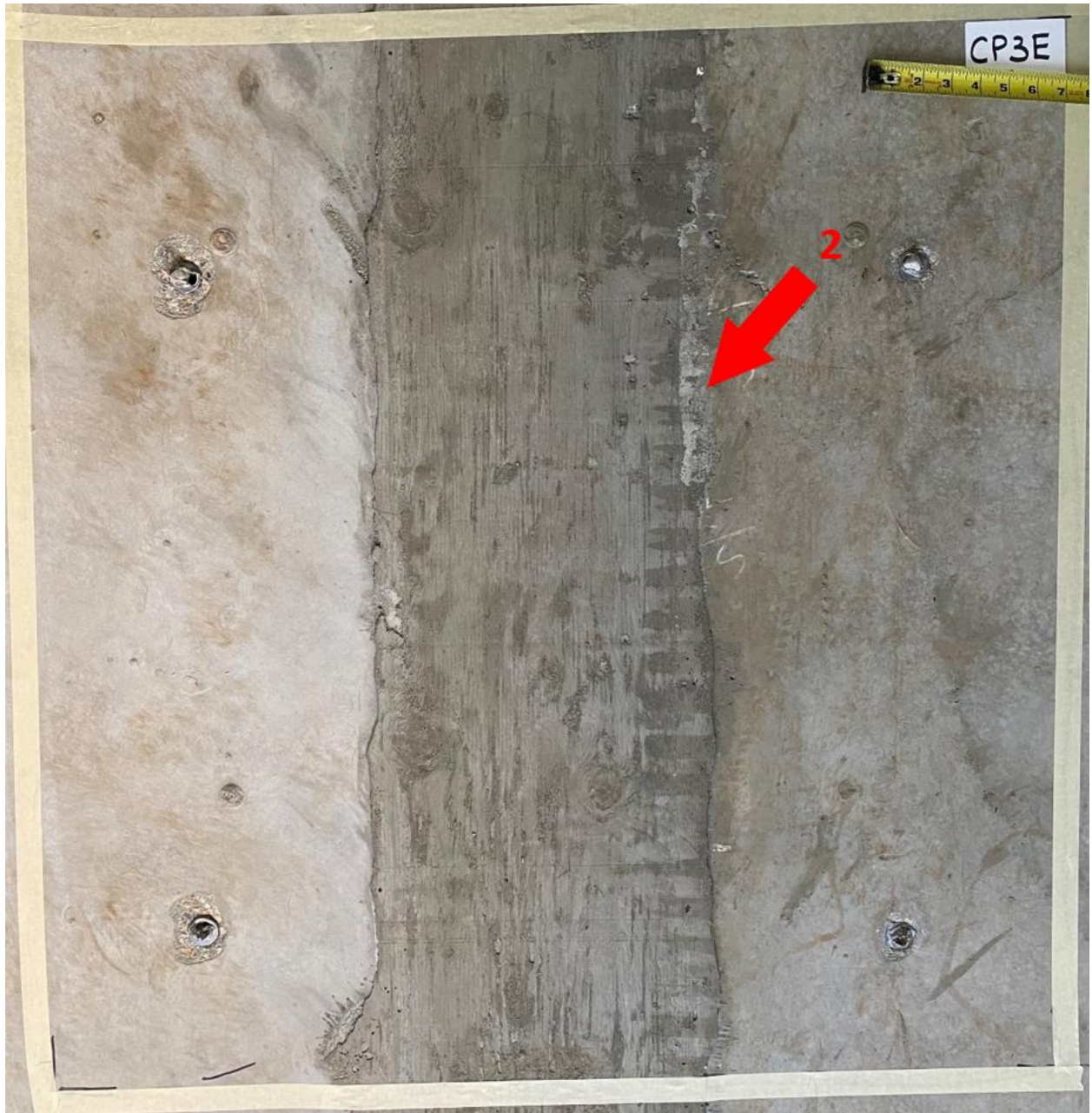
Figure C-15 View of section CP3E, August 27, 2020
