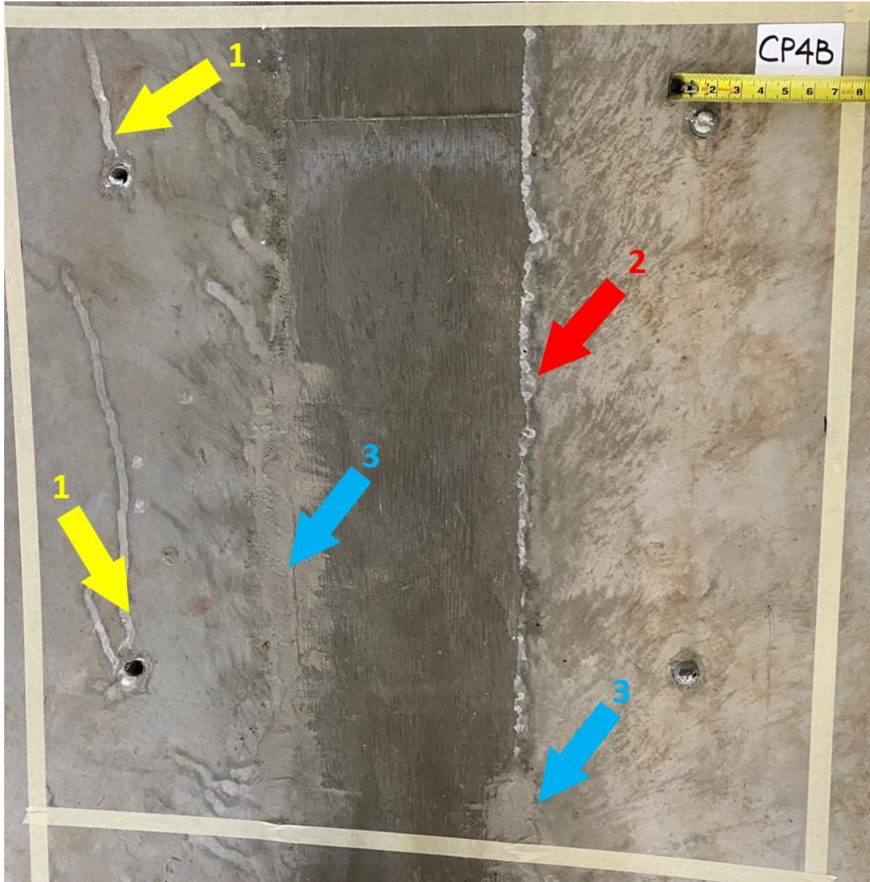
Figure C-17 View of section CP4B, August 27, 2020
