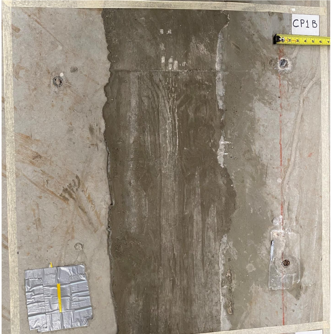
Figure C-22 View of section CP1B, April 5, 2022
