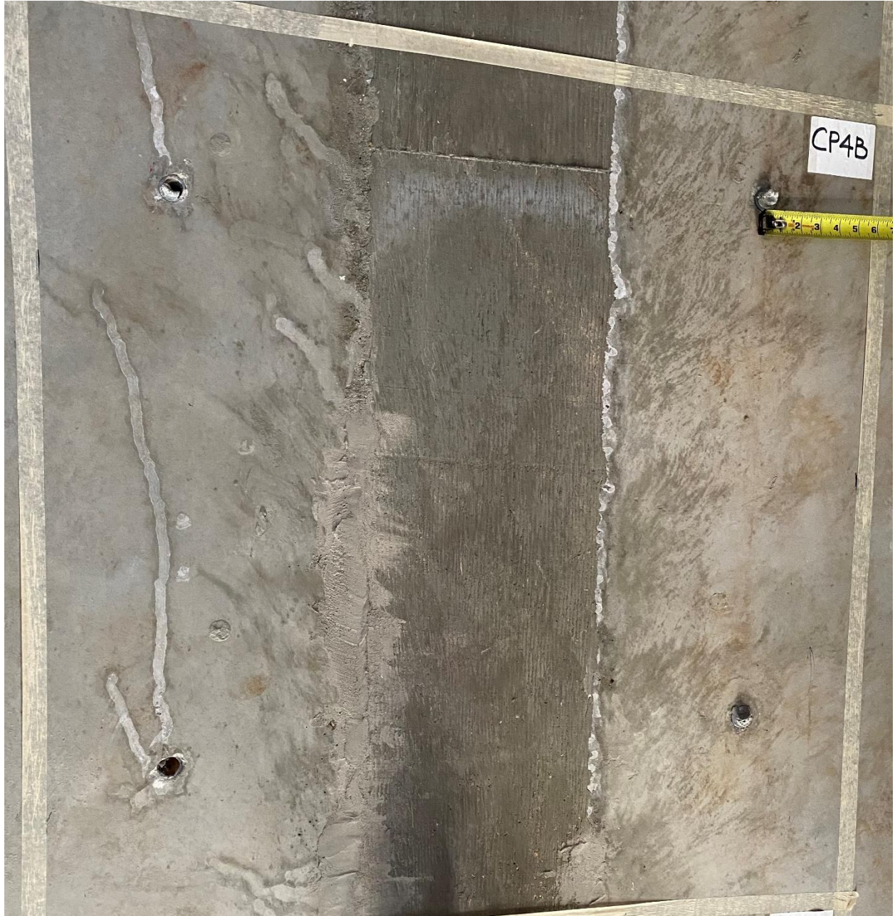
Figure C-37 View of section CP4B, April 5, 2022
