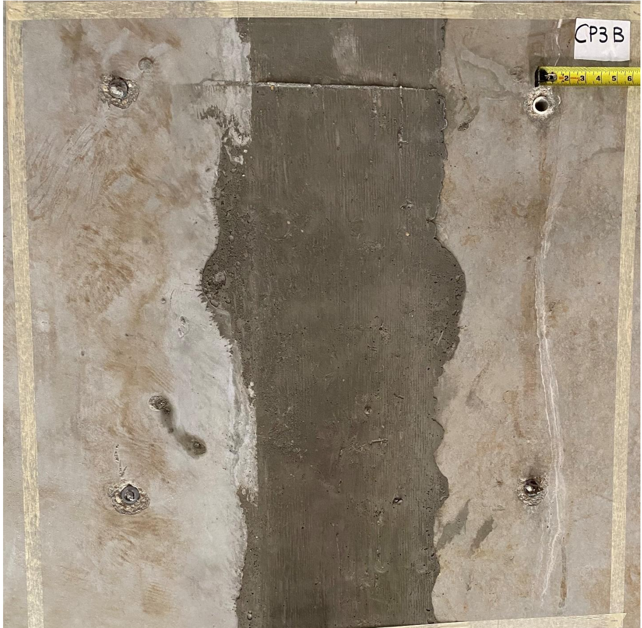
Figure C-32 View of section CP3B, April 5, 2022
