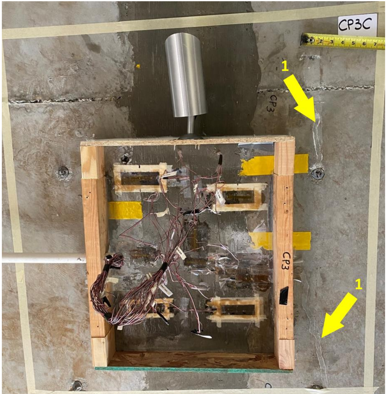
Figure C-13 View of section CP3C, August 27, 2020
