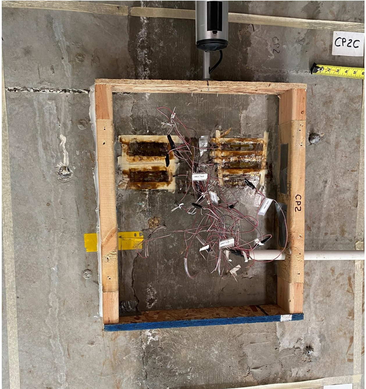
Figure C-28 View of section CP2C, April 5, 2022
