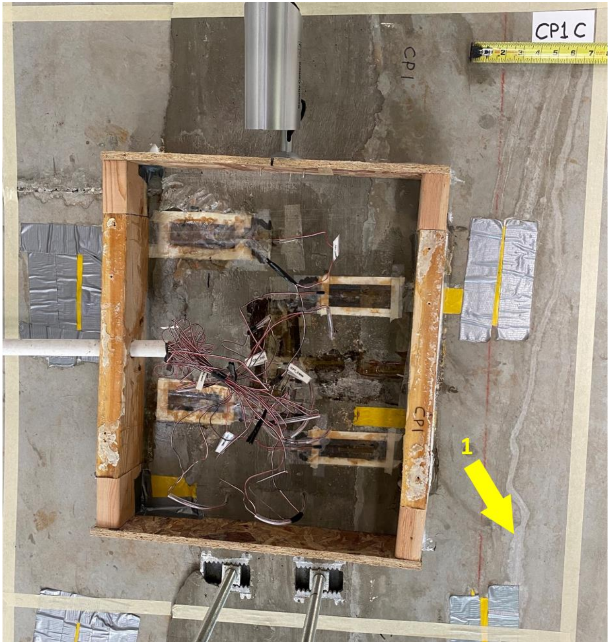
Figure C-3 View of section CP1C, August 27, 2020
