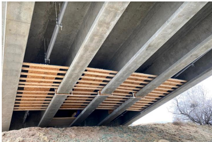
Figure 2-2 Installed access platform
