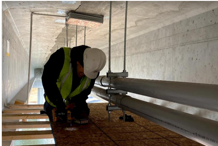
Figure 2-1 Access platform installation
