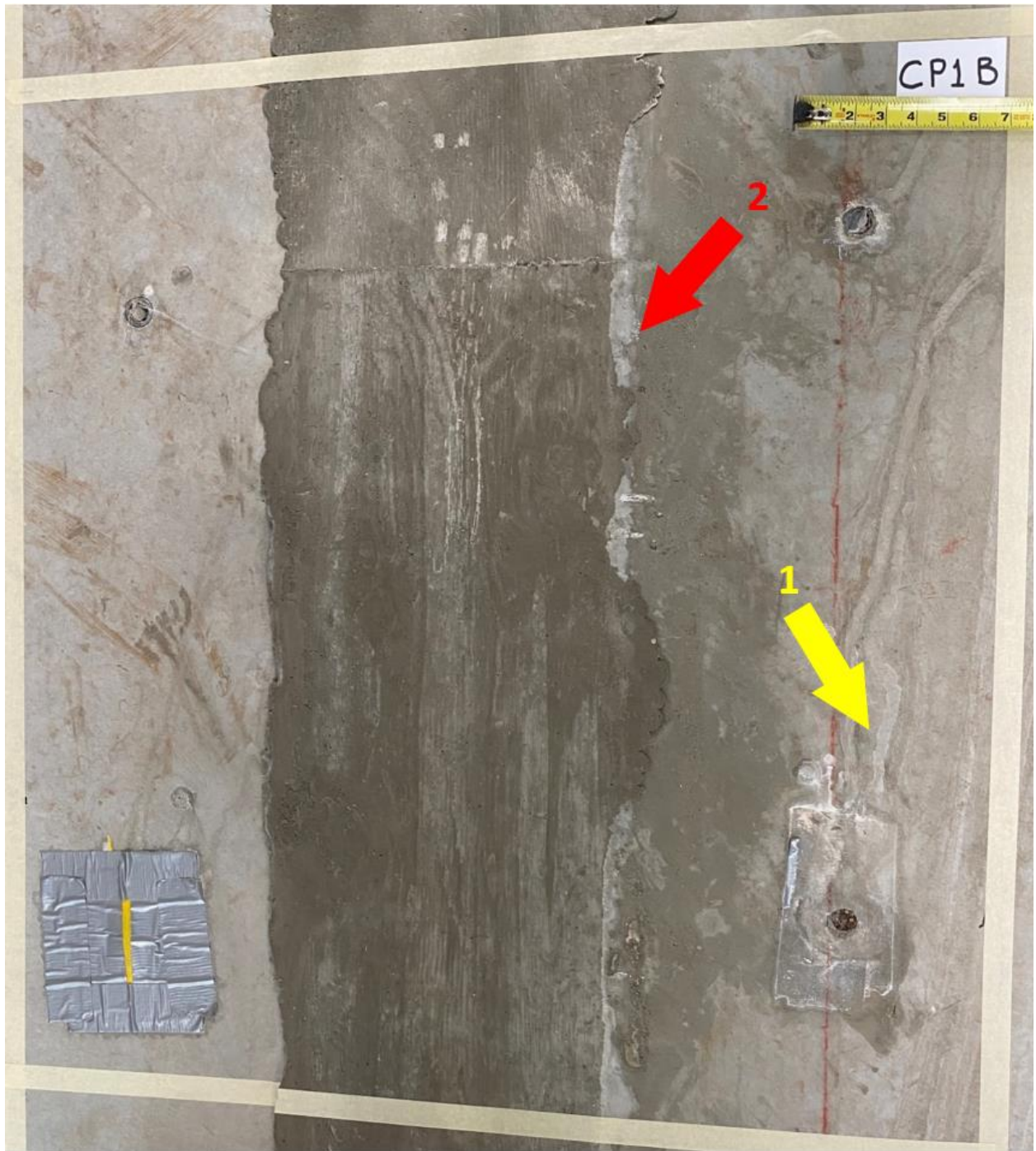
Figure C-2 View of section CP1B, August 27, 2020
