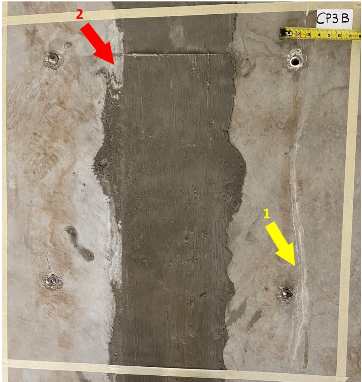
Figure C-12 View of section CP3B, August 27, 2020
