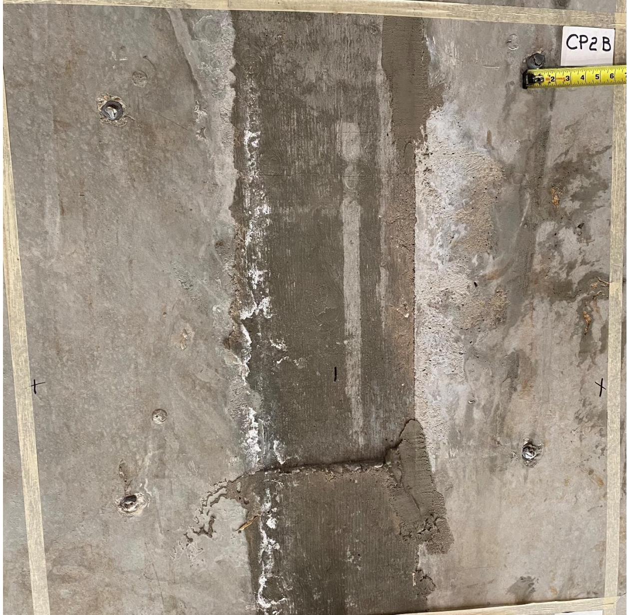
Figure C-27 View of section CP2B, April 5, 2022
