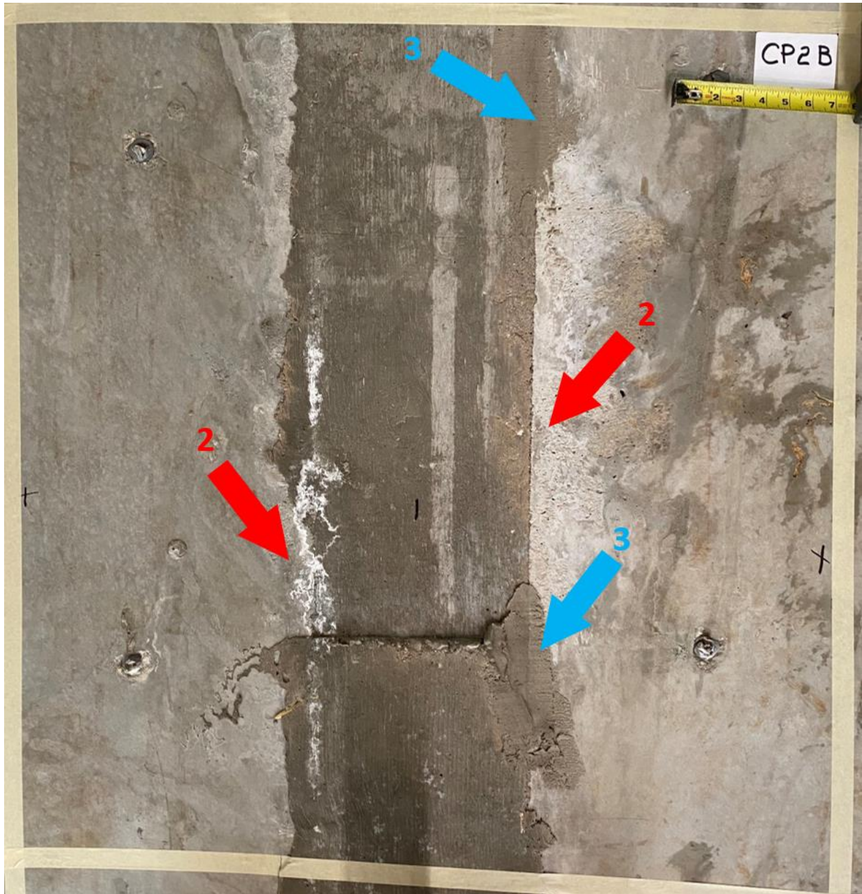
Figure C-7 View of section CP2B, August 27, 2020
