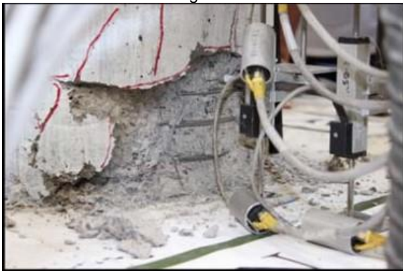
Damage State IV (6.67%)
