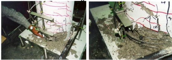
Damage State II
