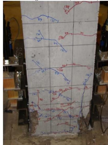
Damage State III (3.51%)
