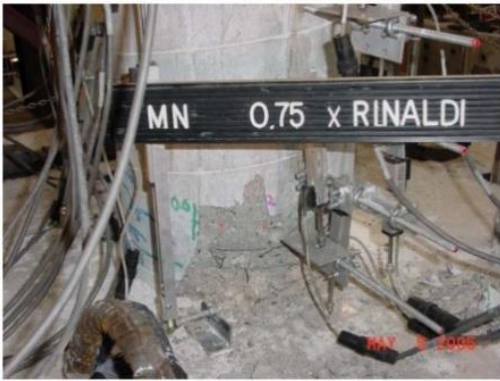
Damage State IV (6.52%)
