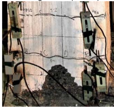
Damage State III (3.53%)
