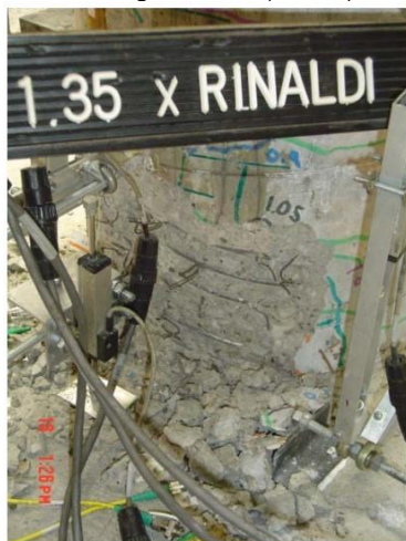
Damage State IV (7.86%)
