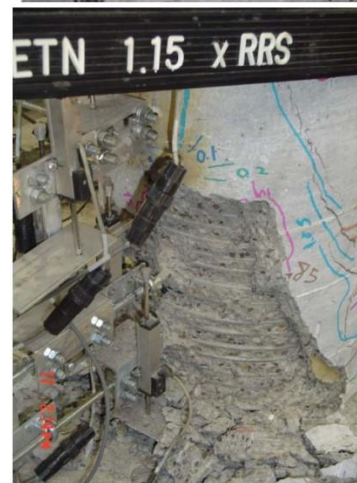
Damage State V-VI (16.83%, 16.83%)
