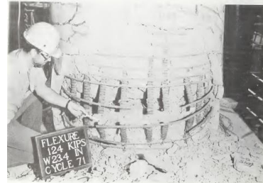
Damage State V (5.88%)
