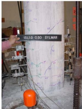
Damage State II (1.72%)
