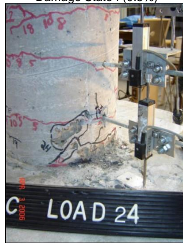
Damage State III (3%)
