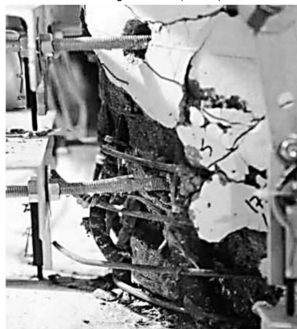
Damage State V (6.0%)
