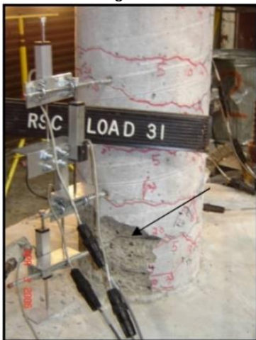
Damage State IV (4%)
