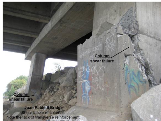
(d) Juan Pablo II Bridge Damage in the 2010 Maule EQ, Built in 1974 (Yashinsky et al., 2010)
