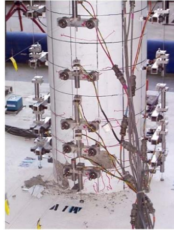
Damage State III (5.07%)
