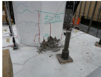
Damage State III (4.42%)
