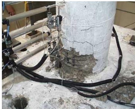
Damage State V-VI (8.19%)
