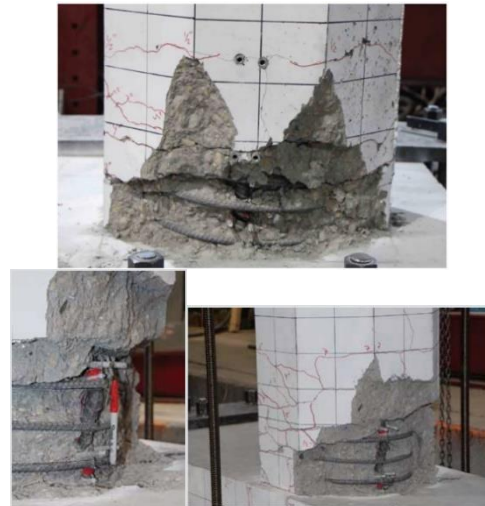
Damage State VI (7.95%, 10%, 10%)
