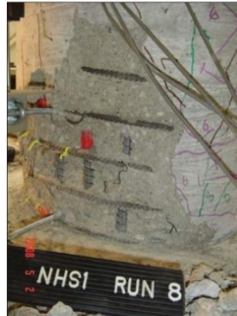
Damage State V (6.87%)
