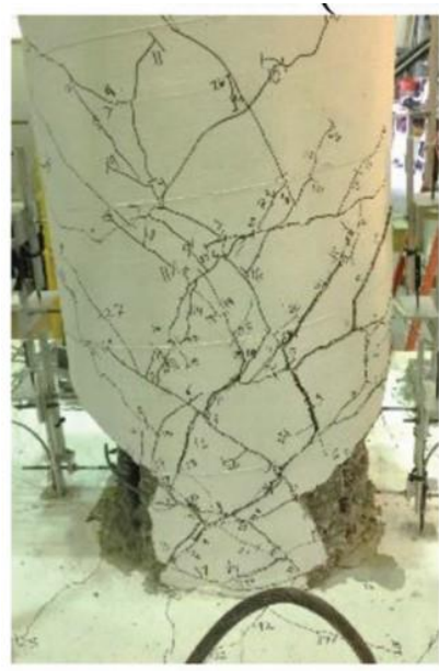
Damage State VI (6%)
