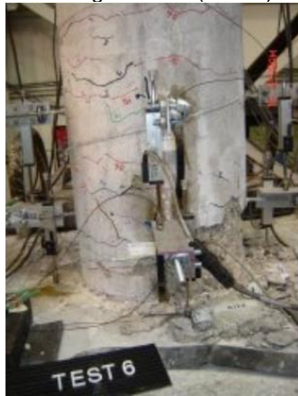
Damage State IV (2.82%)
