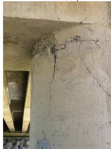
(h) Bridge 2401 Damage at Column Top in the March 2020 Puerto Rico EQ Built in 1996 (Photo by Dr. Manuel Coll)
