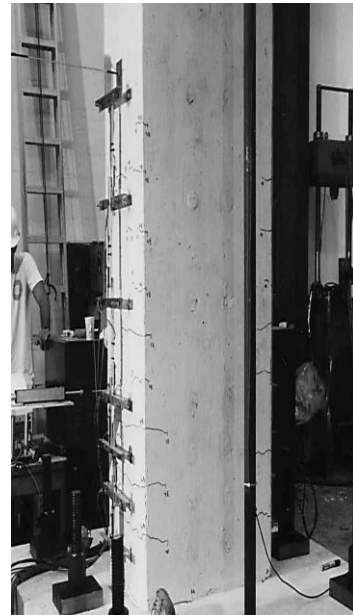
R-5 Column from Hose and Seible (1999) Photo at Drift Ratio: 0.125% Column Height = 144 in. Side Dimension = 28.7 in. by 19.25 in.
