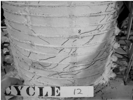
Damage State II (4.75%)
