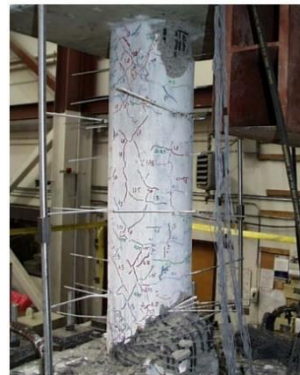
Damage State VI (6.67%)
