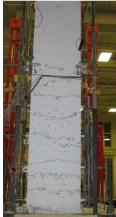
Damage State II (0.642%)
