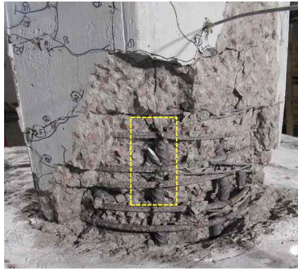
Cast-in-Place Column by Sjurseth (2021) Photo at Drift Ratio: 10.0%; Bar Fracture Column Height = 96 in. Side Dimension = 24 in.
