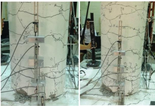
Damage State II (3%, 4%)
