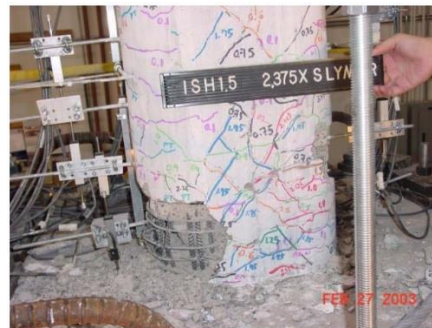
Damage State V (6.67%) & VI (7.29%)
