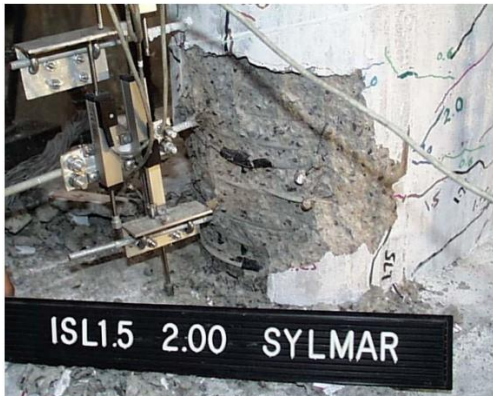
Damage State IV (7.57%)
