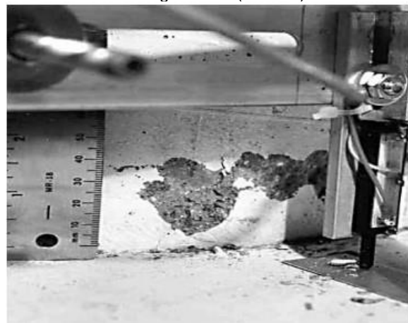
Damage State III (2.53%)
