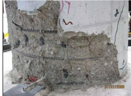
Damage State V (6.17%)
