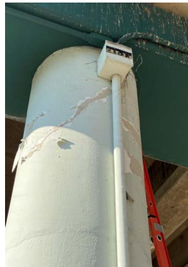
(j) Bridge 0729 Damage at Column Top in the Feb. 2020 Puerto Rico EQ, Built in 1961 (Photo by Dr. Manuel Coll)
