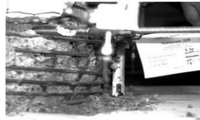
Damage State III
