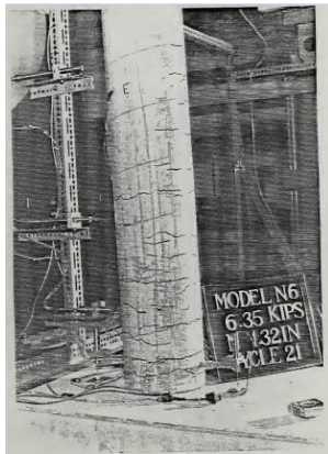
Damage State II (2.24%)
