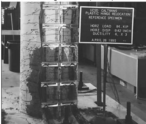
Damage State IV (6.54%)
