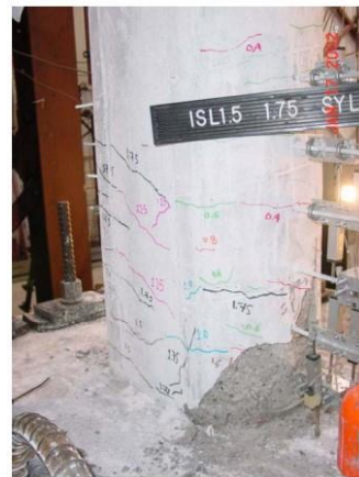
Damage State III (5.36%)
