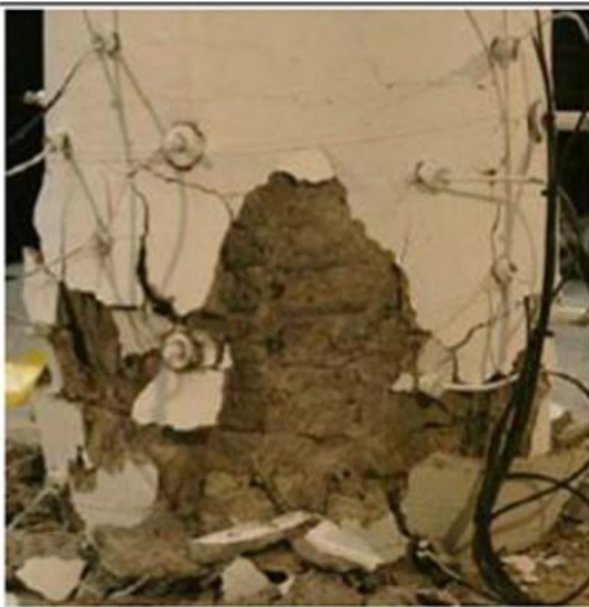
Damage State IV (3.9%)
