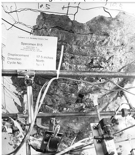
Damage State IV (9.11%)
