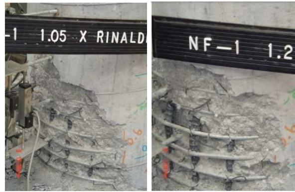
Damage State V (11.82%) & VI (13.3%)
