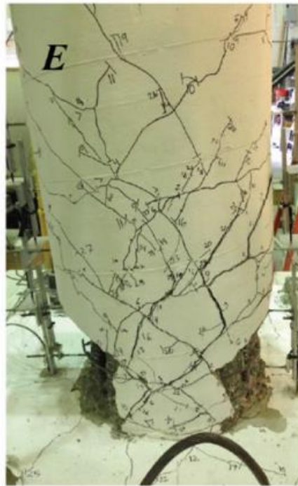
(h) CIP25: failure (6% drift)
