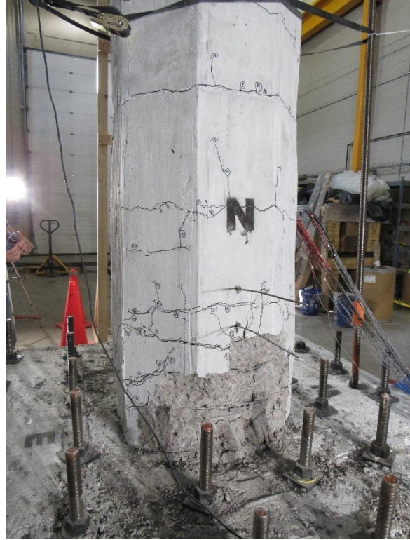
Cast-in-Place Column by Sjurseth (2021) Photo at Drift Ratio: 5.0% Column Height = 96 in. Side Dimension = 24 in.
