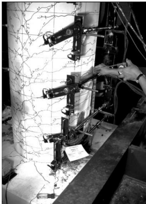
Damage State IV (2.78%)
