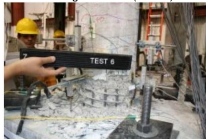
Damage State V (7.6%)
