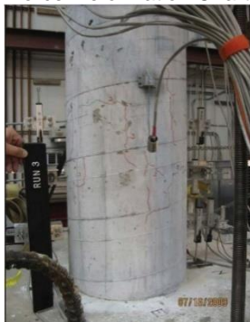
Damage State II (1.53%)
