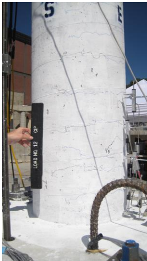
Damage State II (0.75%)
