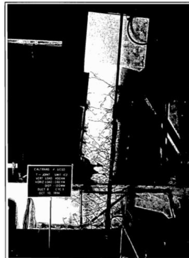
Damage State VI (6.56%)
