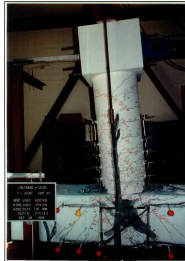
Damage State VI (7.48%)
