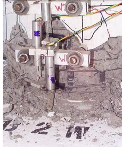
Damage State III
