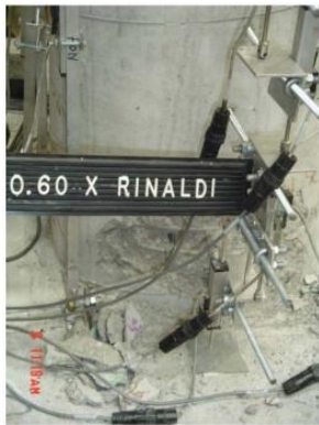
Damage State IV (6.92%)
