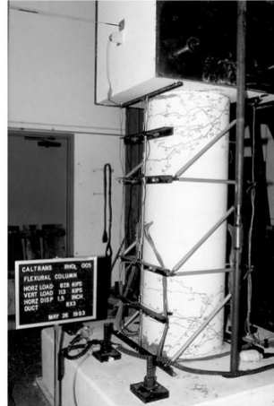
Damage State III (1.67%)
