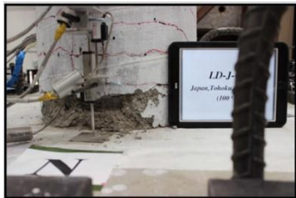
Damage State III (6.26%)
