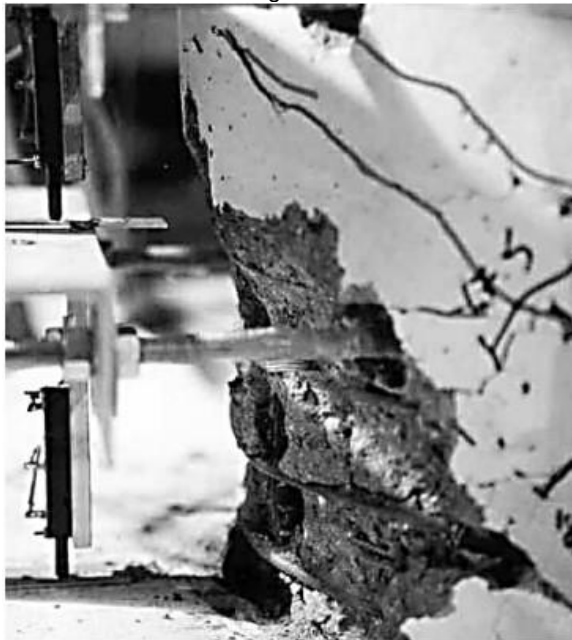
Damage State IV (5.0%)
