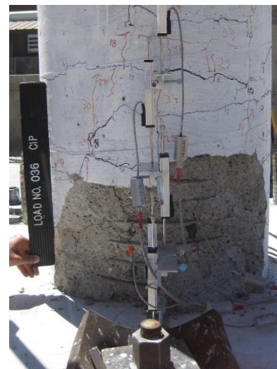
Damage State V (6%)
