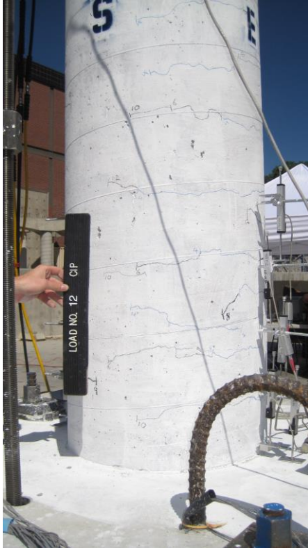
Cast-in-Place Column by Haber et al. (2013) Photo at Drift Ratio: 0.75% Column Height = 108 in. Diameter = 24 in.
