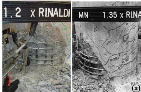
Damage State V (11.92%) & VI (14.4%, 14.4%)
