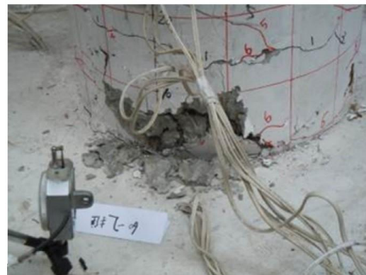
Damage State III (3.75%)
