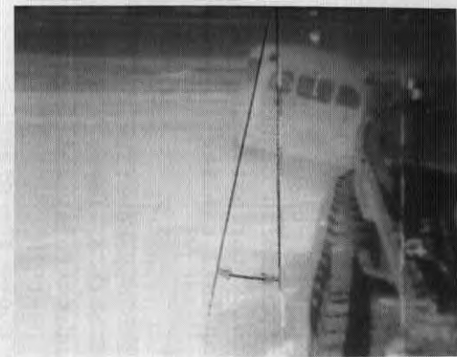
(c) Collapsing ring bridge railing
