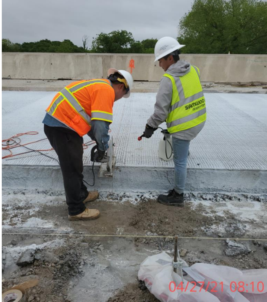
Figure 5.19 Sawcut operation
