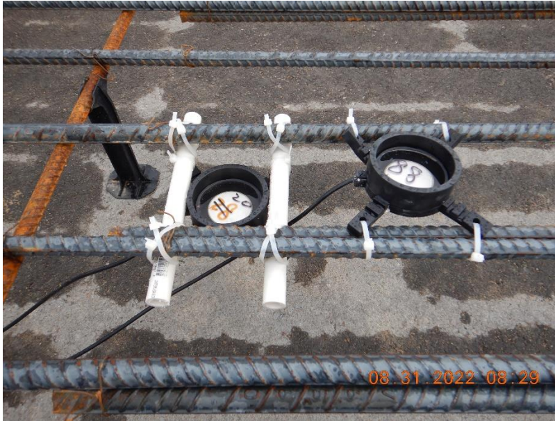
Figure 5.6 REBEL Sensor and its typical installation
