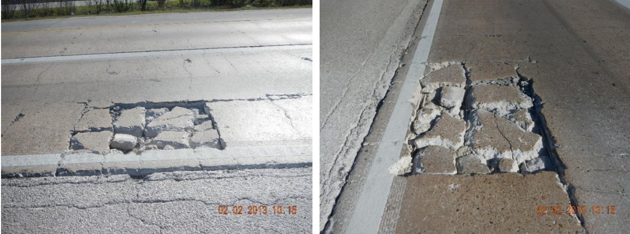
Figure 2.8- (a) Punchout distress on Loop 610 (left); (b) Punchout on Loop 610 (right)
