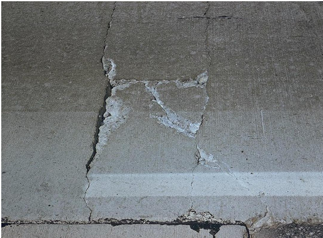
Figure 2.2 CRCP distress presented as a punchout in several documents
