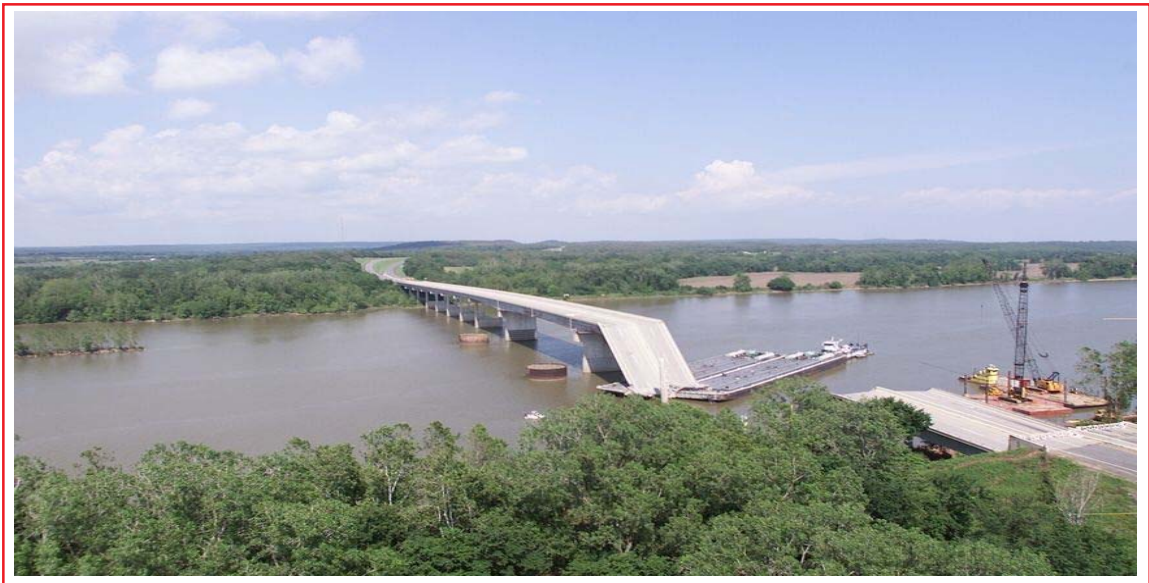
Figure 1. May 2002 Barge Impact with I-40 Webbers Fall Bridge (Provided by Oklahoma DOT)
