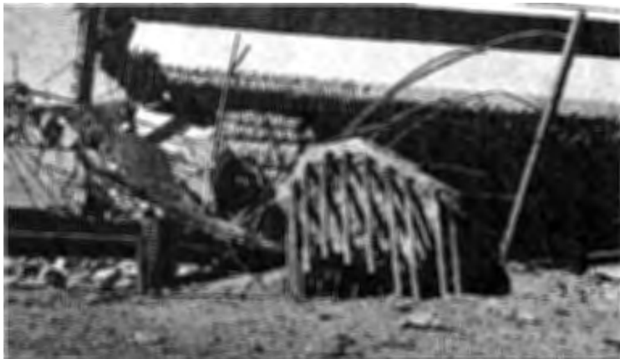
Figure 36.- Route 5/210 Separation and Overhead bridge. Bottom of pier 5 column at construction joint. Reinforcing bars were pulled cleanly out of the CIDH pile shaft due to bond failure. California Division of Highways, Bridge Department photograph.
