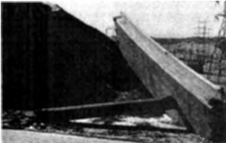
Figure 34.- Route 5/210 Separation and Overhead bridge. Portion of collapsed superstructure and pier 2 column. Abutment 1 (south abutment) is at top of embankment. Note that the right wingwall is completely sheared off whereas the left wall is undamaged. California Division of Highways, Bridge Department photograph.
