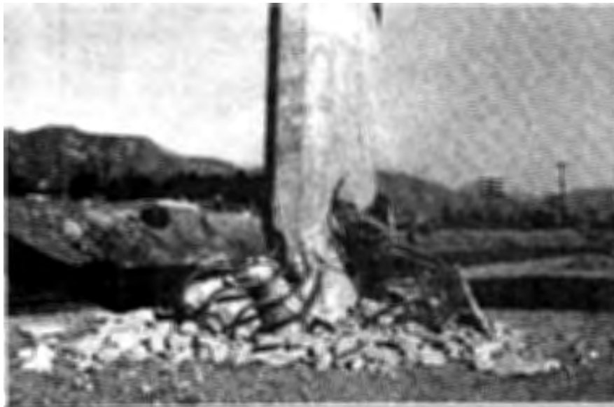
Figure 21.- San Fernando Road Overhead bridge. Closeup of column base. Note flareout of vertical reinforcing bars. California Division of Highways. Bridge Department photograph.
