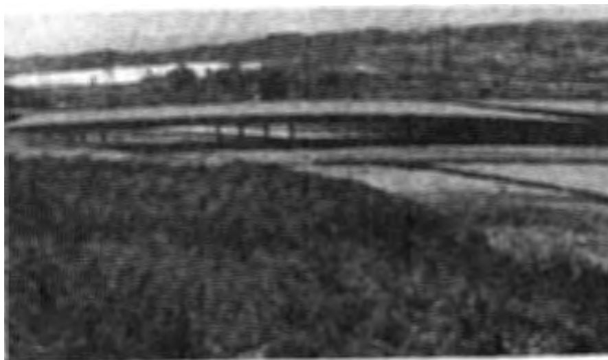
Figure 27.- Northwest Connector Overcrossing bridge. Note that the superstructure has dropped off the seat of abutment 1 in the right portion of the photograph. California Division of Highways, Bridge Department photograph.
