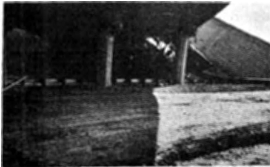
Figure 29.- Northwest Connector Overcrossing bridge. Bent 4 columns. Note severe crushing of concrete at tops of columns as well as displacements due to superstructure rotation. Note also fallen superstructure of adjacent bridge at right of photo. California Division of Highways, Bridge Department photograph.
