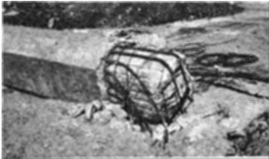
Figure 35.- Route 5/210 Separation and Overhead bridge. Bottom of pier 2 column. Core of column pulled out of pile cap due to bond failure. California Division of Highways, Bridge Department photograph.
