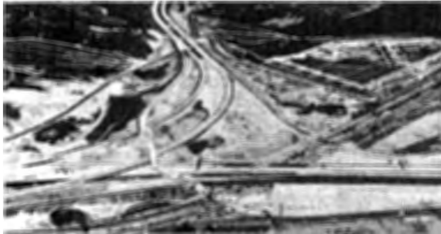
Figure 31.- Route 5/210 Interchange, looking northeast. Route 5 crosses lower portion of photograph and Route 210 approaches the interchange from the top. Note collapsed Separation and Overhead bridge near center of photograph. California Division of Highways, Bridge Department photograph.
