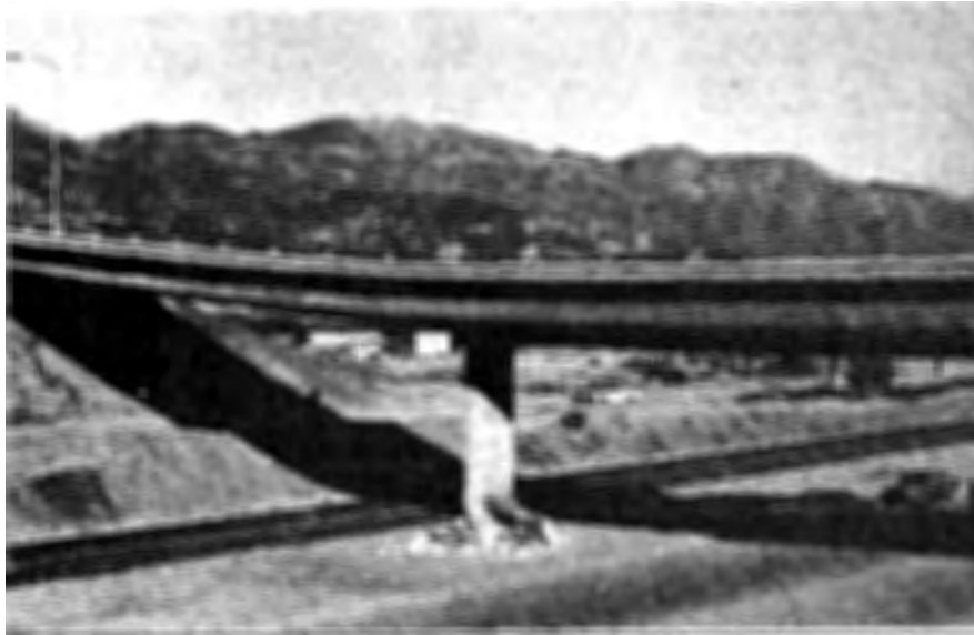
Figure 20.- San Fernando Road Overhead bridge. Damaged column. Note cracks in superstructure on either side of bent cap. California Division of Highways, Bridge Department photograph.
