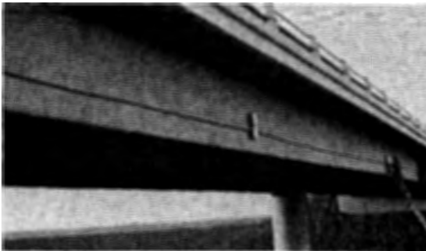
Figure 54.- View southeastward of Meloland overcrossing. Note two pairs of FBA-1 accelerometers, which are encased in metal boxes (fig. 55B). PVC conduit used here to protect interconnect cable found to be highly unsatisfactory due to thermal expansion and contraction.
