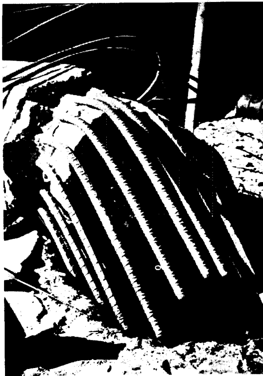
FIGURE B-3: COLUMN FAILURE RTE 210/5 SEPARATION AND O.H.
