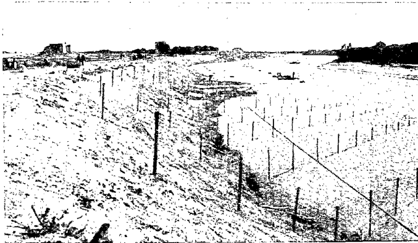
FIGURE 17. WIRE FENCE SPURS (SOURCE: U.S. ARMY CORPS OF ENGINEERS, 1981)
