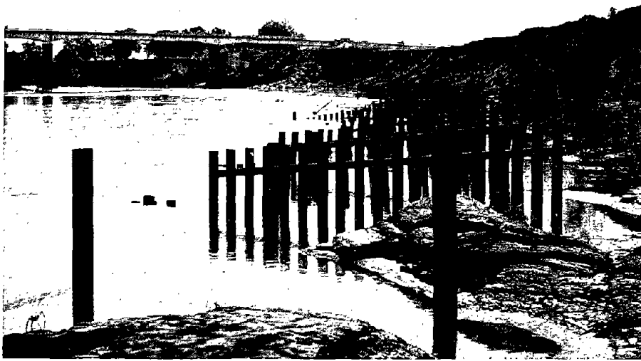
FIGURE 14. HENSON TYPE SPUR JETTY. BARZOS RIVER NEAR ROSHARON, TEXAS.
