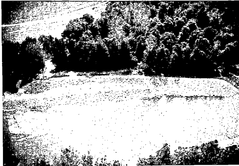
FIGURE 24. ROCK RIPRAP SPUR, LOYALSOCK CREEK NEAR MONTOURSVILLE, PA. (COURTESY PENNSYLVANIA DEPT. OF TRANSPORTATION, DISTRICT 3-0)
