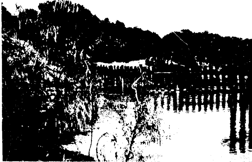
FIGURE 61. HENSON SPUR SHOWING OUTFLANKING.
