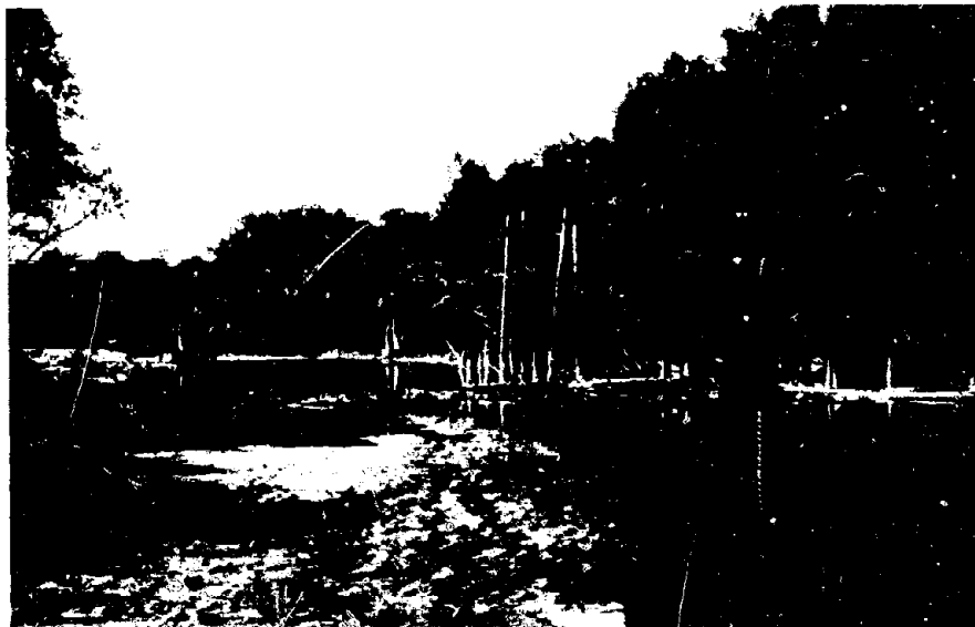
FIGURE 9. TIMBER PILE SPURS; BIG BLACK RIVER AT DURANT, MISSISSIPPI.
