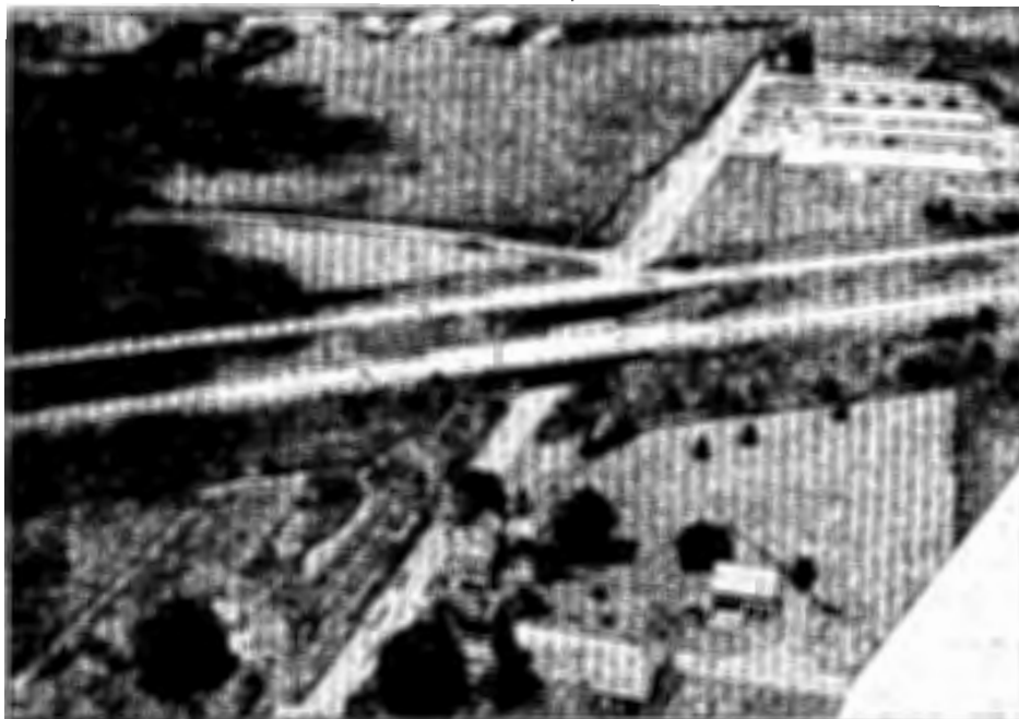
Figure 18. Aerial view of bridges over Van Buren Road.
