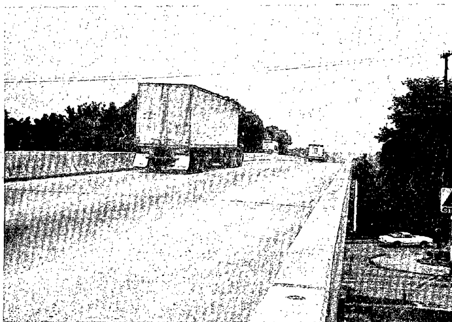
Figure 7. Looking east over the EB Bridge.
