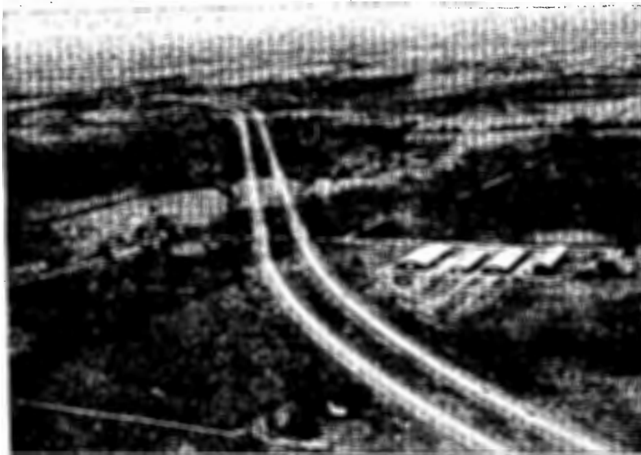
Figure 17. Aerial view of Route 33 looking southwest.
