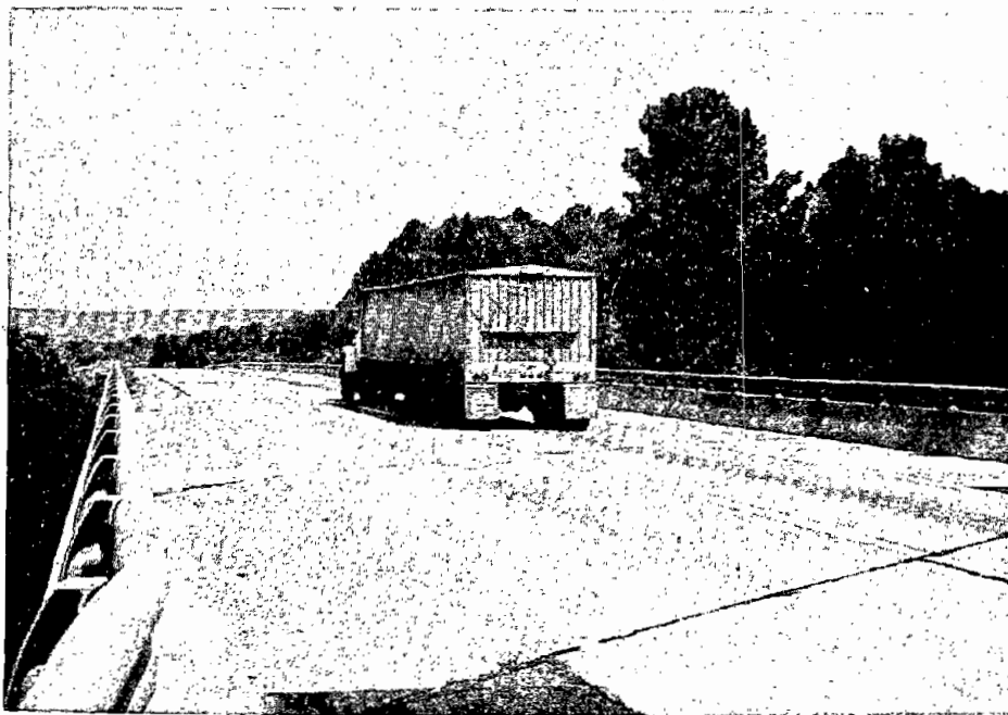
Figure 29. Looking north over the NB Bridge.
