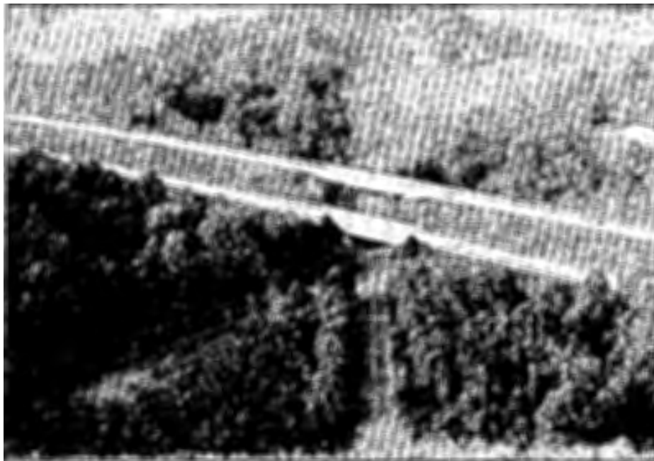
Figure 27. Aerial view of bridges over State Park Road.
