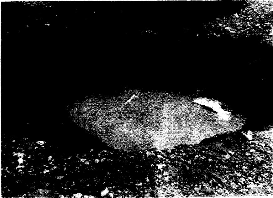
Figure 25 : Ground water rise into a crater following dynamic compaction
