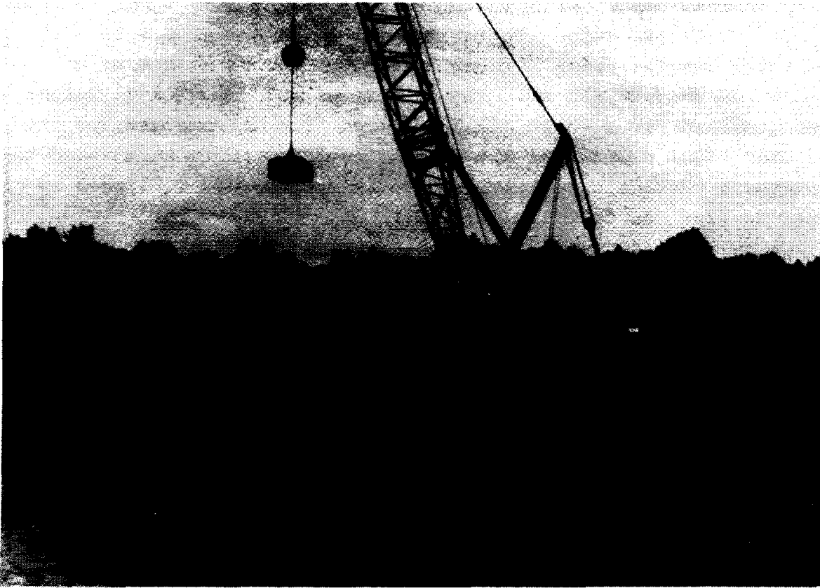
Figure 1 : A 125 ton crawler crane lifting a 15 - tonne weight to a height of 20 meters
