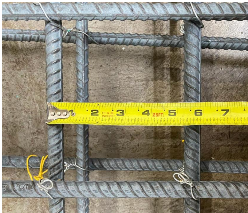
Figure 78. Photo. Checking reinforcement spacing of 6 in.
