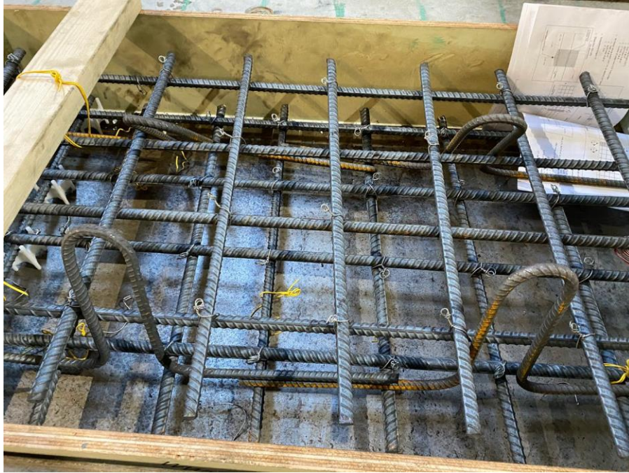
Figure 81. Photo. Hooked No. 4 bars placed inside reinforcement cage for lifting purposes.
