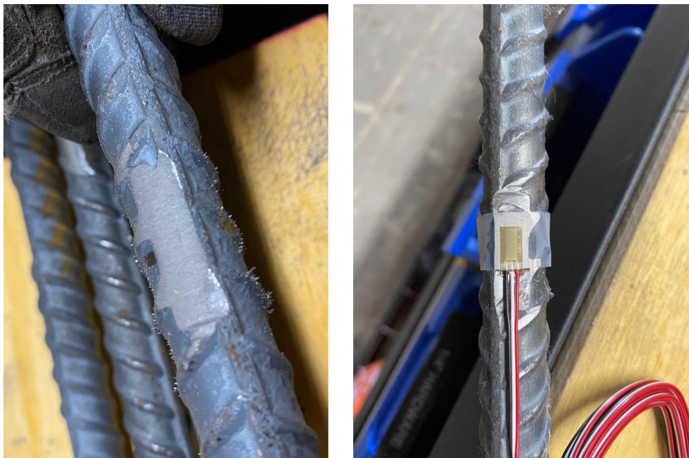
Figure 74. Photo. Surface preparation for strain gauge attachment.
