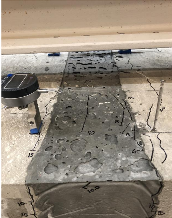
Figure 133. Photo. Locations of cracks within UHPC marked at 15 kips.
