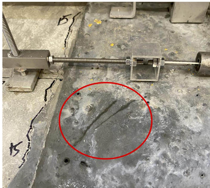
Figure 104. Photo. Cracks on the top face of UHPC joint at circled in red.
