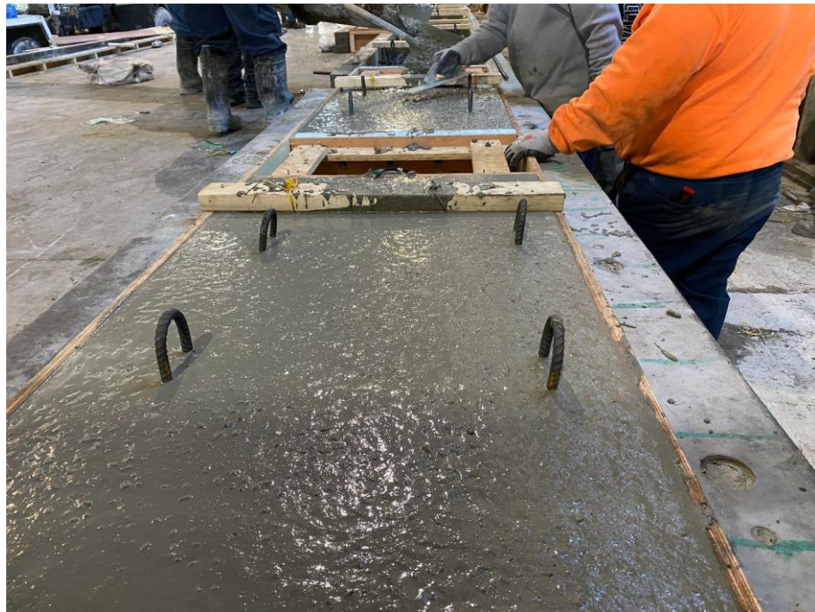
Figure 83. Photo. Deck panel specimens being cast.
