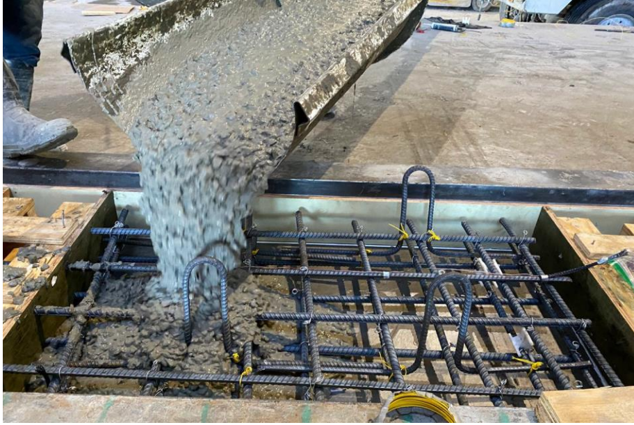
Figure 82. Photo. Deck panel specimen being cast with ready-mix truck.
