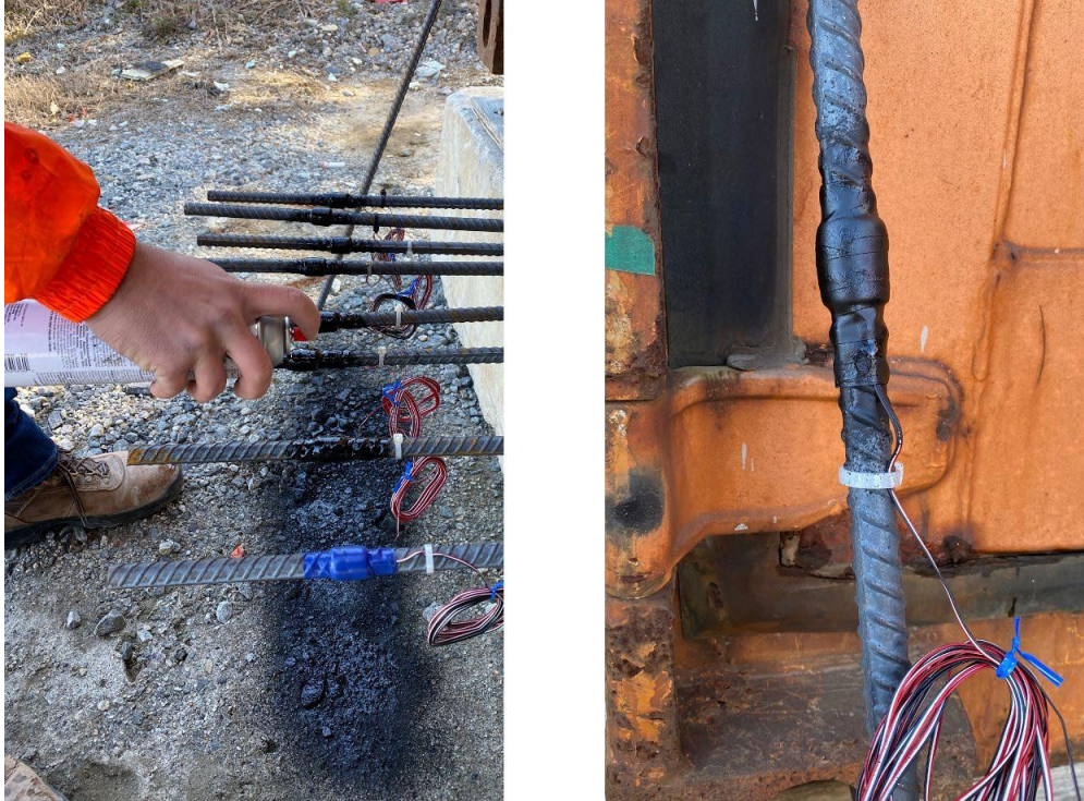
Figure 76. Photo. Spray-on sealant being applied to provide protection against water.
