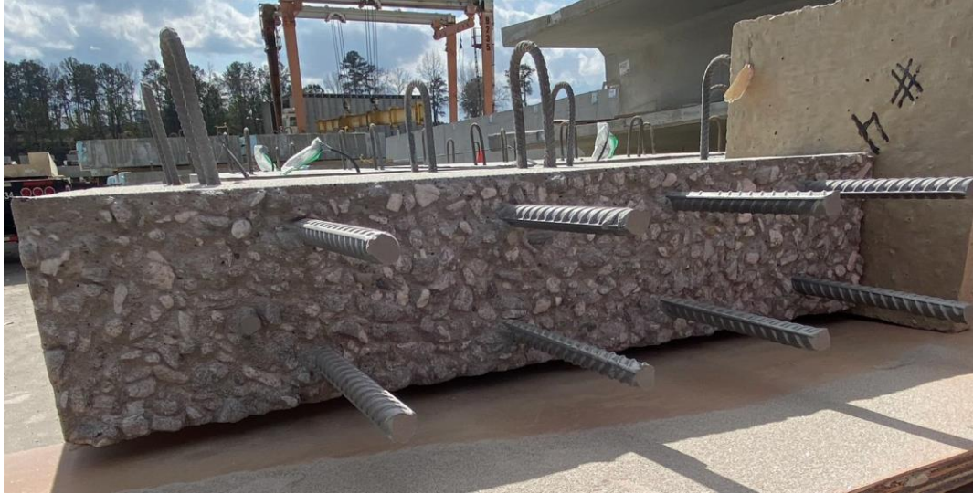
Figure 88. Photo. Sand-blasted surface.
