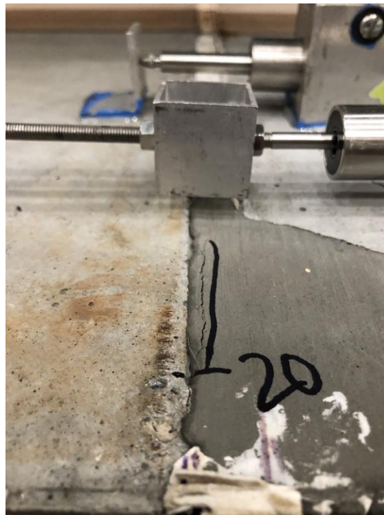
Figure 151. Photo. Crack within UHPC joint occurring at 20 kips of applied load.
