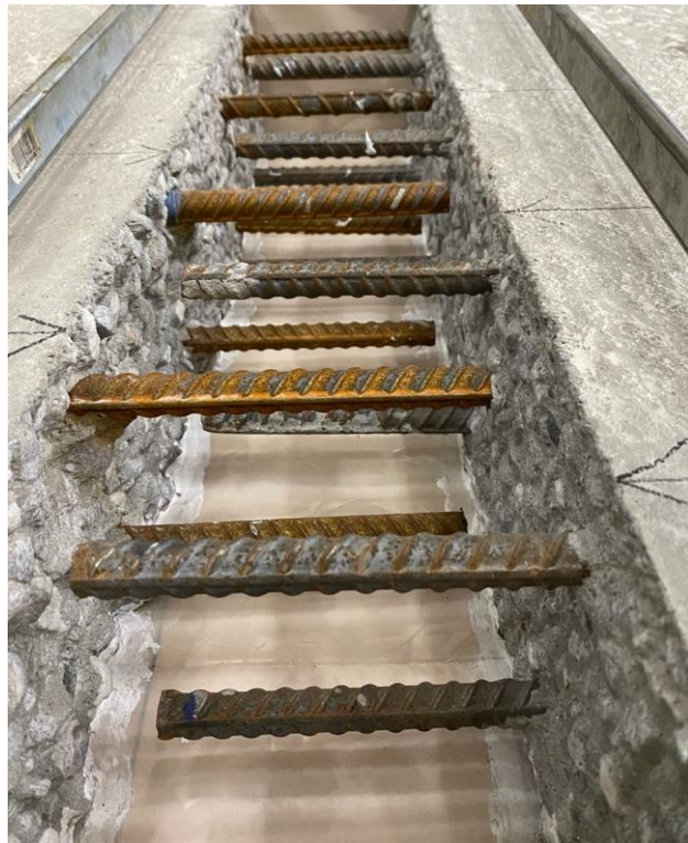
Figure 91. Photo. Non-contact lap splice in the joint region.
