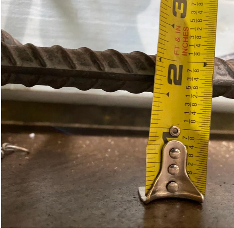
Figure 79. Photo. Checking bottom cover of steel reinforcement in a specimen.
