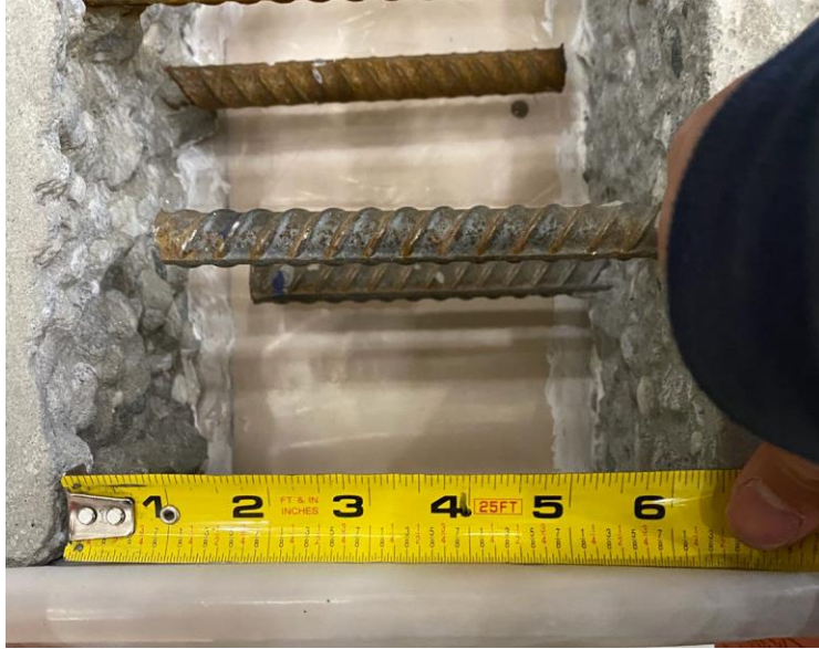
Figure 90. Photo. 6 in. wide joint region between two deck panels.
