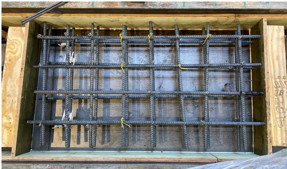
Figure 80. Photo. Reinforcement cage of a 28 in. by 48 in. by 9 in. specimen.
