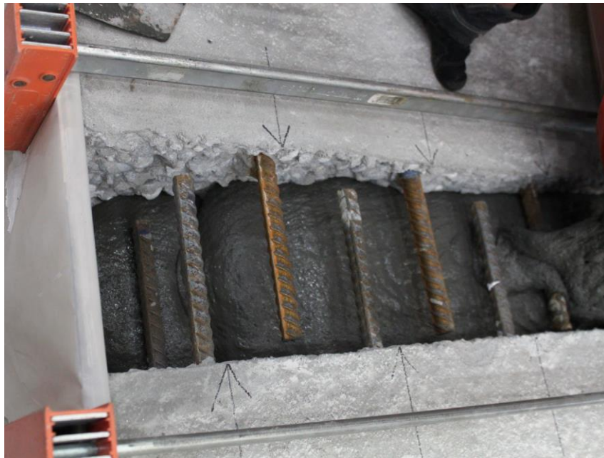
Figure 94. Photo. Close-up of UHPC joint pour.
