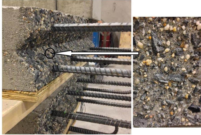
Figure 15. Photo. EA surface of a precast concrete deck. (40)
