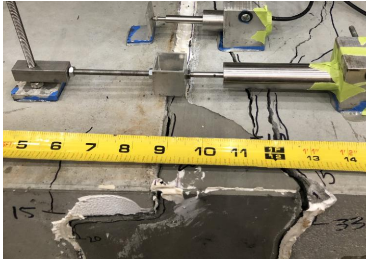
Figure 163. Photo. Large cracks along damaged shear key of precast concrete panel at failure.
