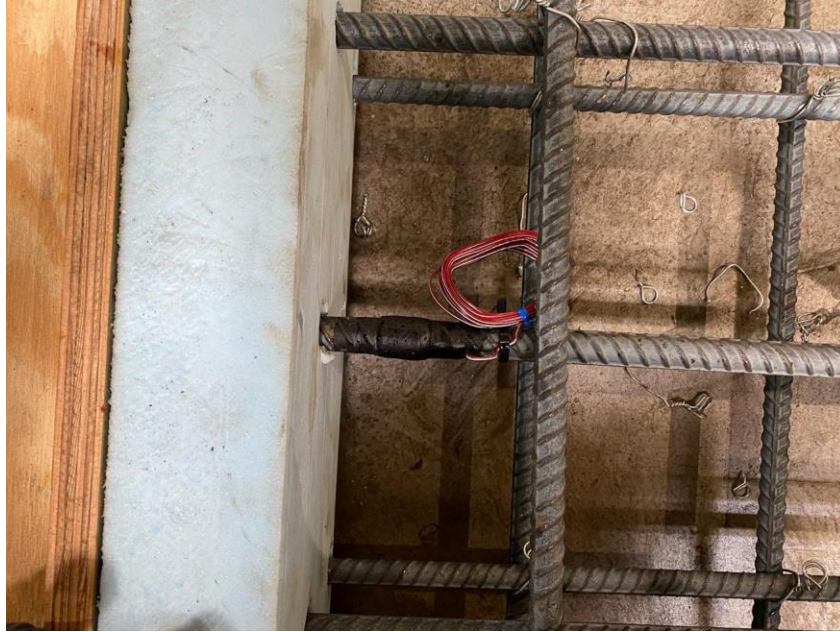
Figure 77. Photo. No. 5 bar with a strain gauge inside reinforcement cage.
