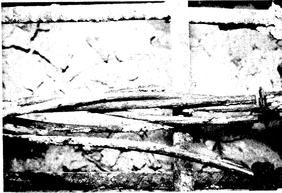
Figure 29. Appearance of interior of tendon bundle in north repair area, slab 2, after 100 exposure cycles.
