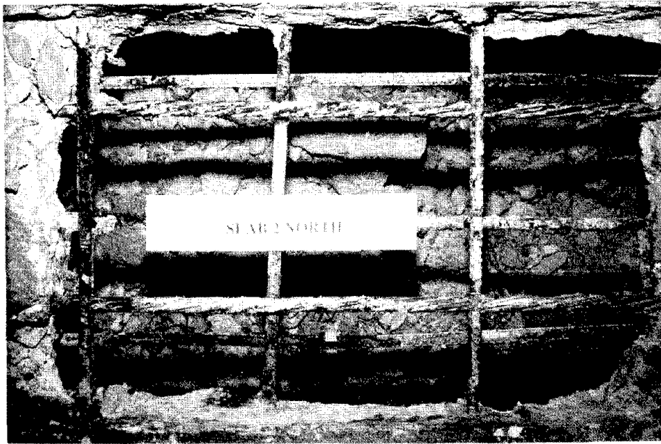
Figure 27. Appearance of uncovered tendons and reinforcing steel in north repair area, slab 2, after 100 exposure cycles.
