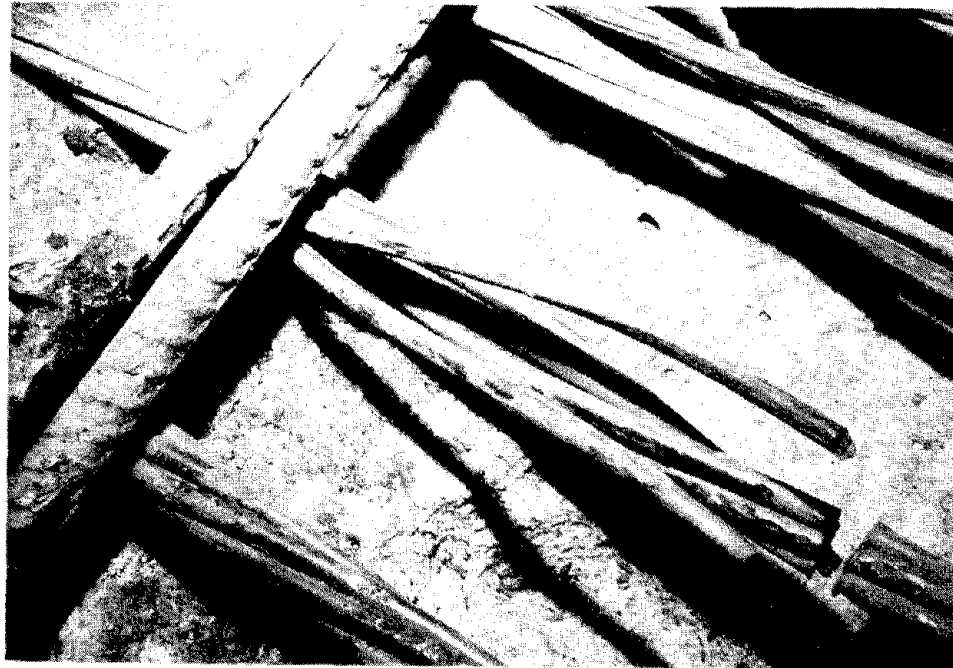
Figure 52. Appearance of interior of tendon bundle in south repair area, beam 3, after 100 exposure cycles.
