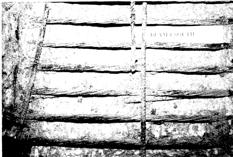
Figure 42. Appearance of uncovered tendons and reinforcing steel in south repair area, beam 1, after 100 exposure cycles.
