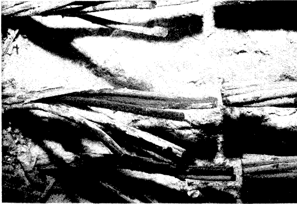
Figure 61. Appearance of interior of tendon bundle in north repair area, pile 2, after 215 weeks of tidal cycling.
