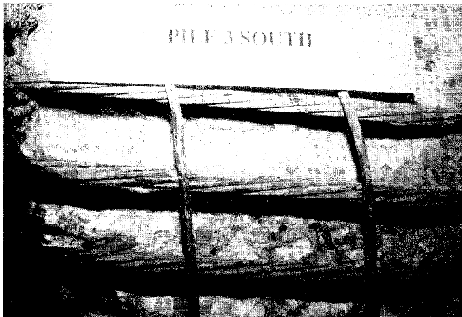
Figure 64. Appearance of uncovered tendons and reinforcing steel in south repair area, pile 3, after 215 weeks of tidal cycling.
