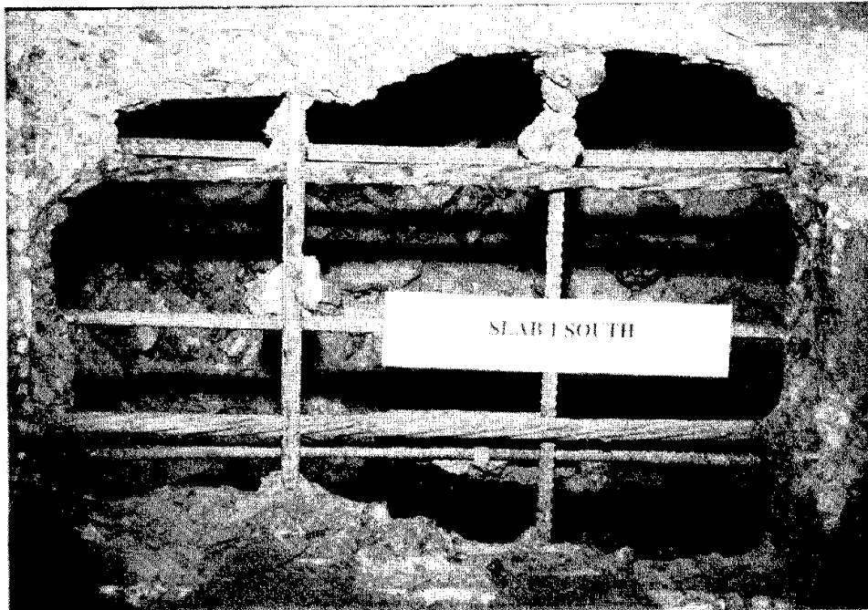
Figure 24. Appearance of uncovered tendons and reinforcing steel in south repair area, slab 1, after 100 exposure cycles.
