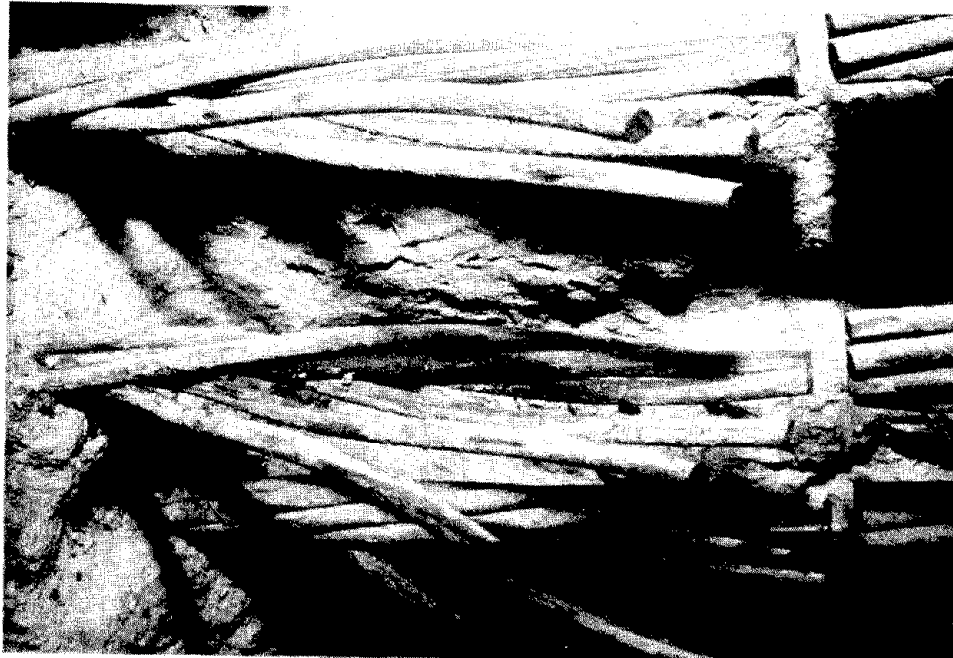
Figure 66. Appearance of interior of tendon bundle in south repair area, pile 3, after 215 weeks of tidal cycling.
