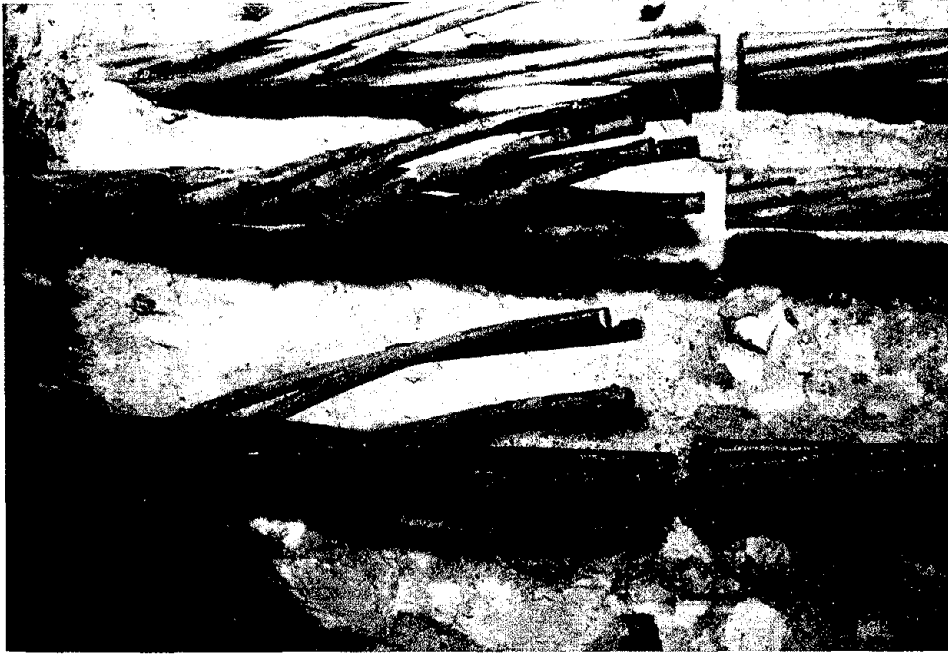
Figure 65. Appearance of interior of tendon bundle in north repair area, pile 3, after 215 weeks of tidal cycling.
