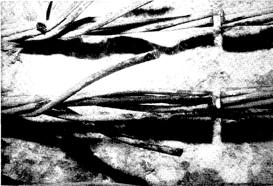
Figure 58. Appearance of interior of tendon bundle in south repair area, pile 1, after 215 weeks of tidal cycling.
