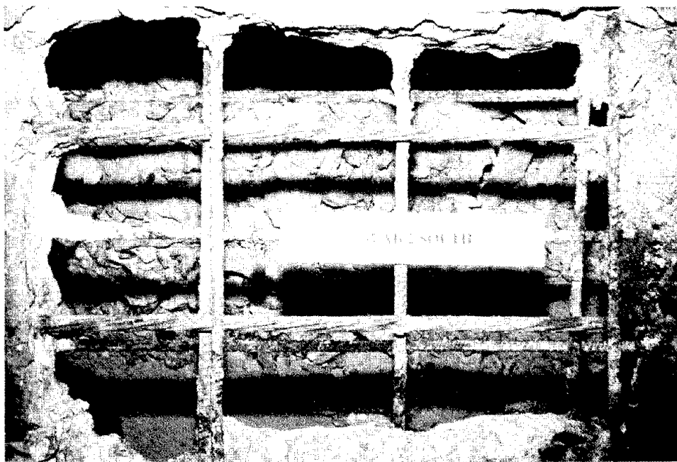
Figure 28. Appearance of uncovered tendons and reinforcing steel in south repair area, slab 2, after 100 exposure cycles.
