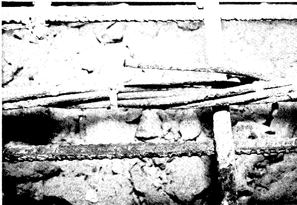
Figure 30. Appearance of interior of tendon bundle in south repair area, slab 2, after 100 exposure cycles.
