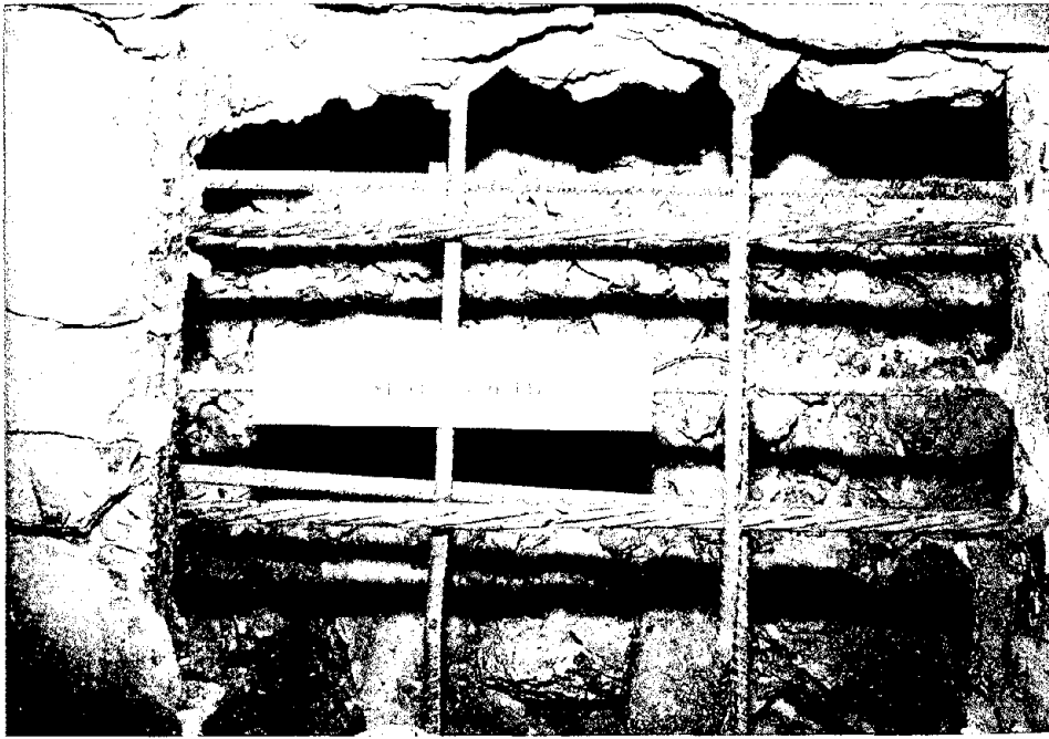
Figure 31. Appearance of uncovered tendons and reinforcing steel in north repair area, slab 3, after 100 exposure cycles.
