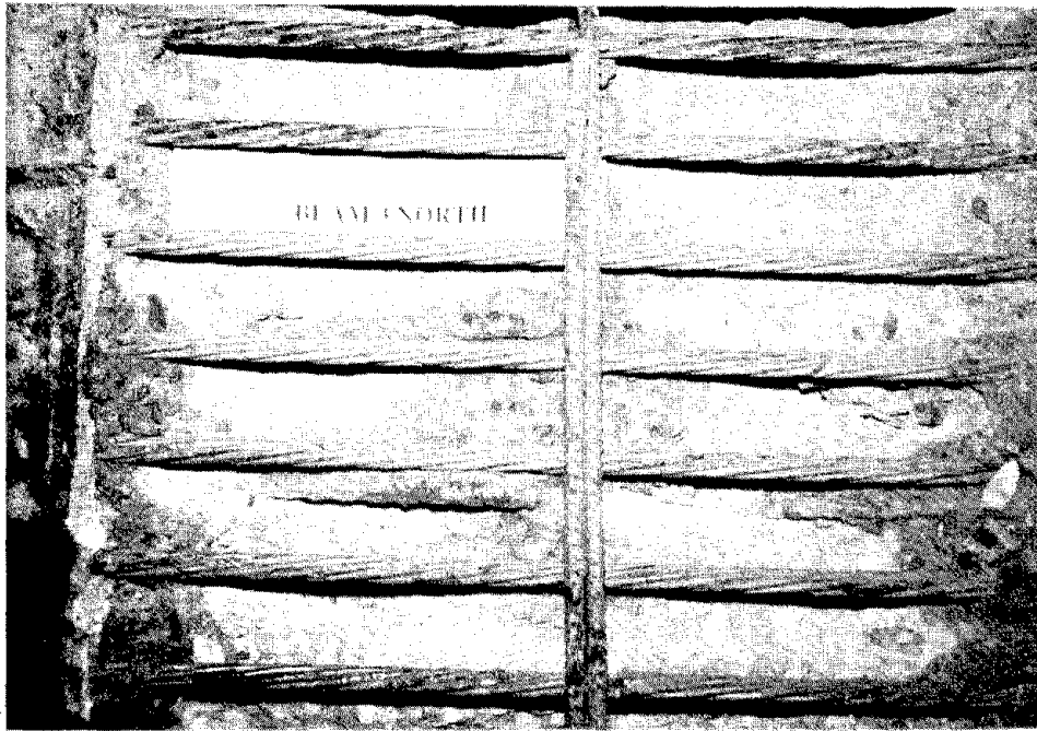
Figure 49. Appearance of uncovered tendons and reinforcing steel in north repair area, beam 3, after 100 exposure cycles.
