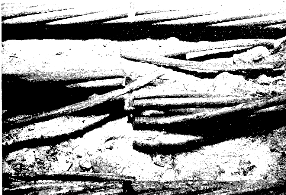
Figure 48. Appearance of interior of tendon bundle in south repair area, beam 2, after 100 exposure cycles.
