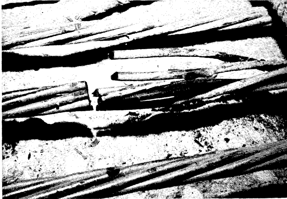
Figure 51. Appearance of interior of tendon bundle in north repair area, beam 3, after 100 exposure cycles.
