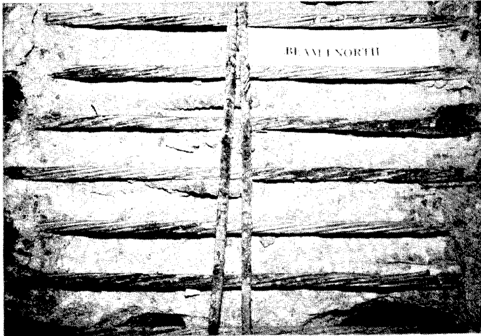
Figure 41. Appearance of uncovered tendons and reinforcing steel in north repair area, beam 1, after 100 exposure cycles.
