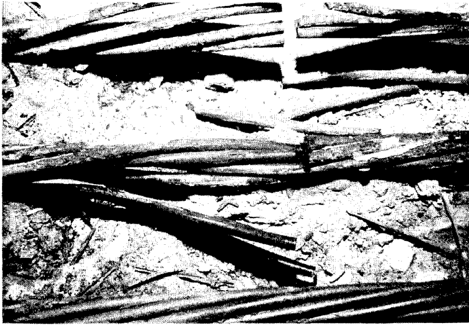
Figure 43. Appearance of interior of tendon bundle in north repair area, beam 1, after 100 exposure cycles.
