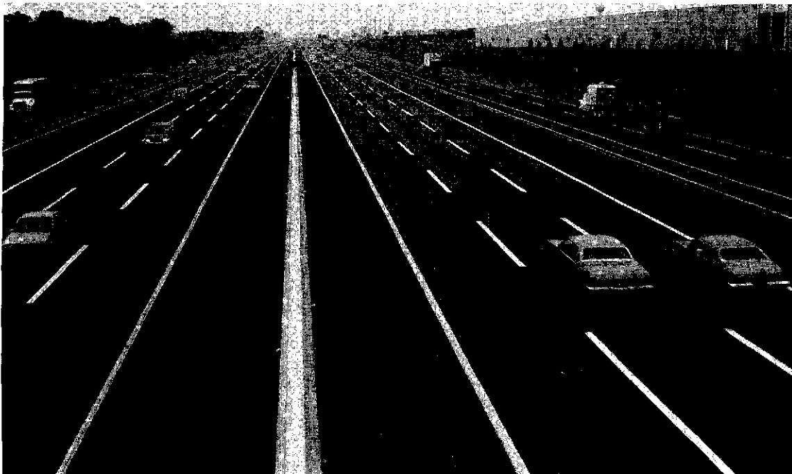
Figure 45. New Jersey Turnpike dual-dual roadway cross section.
