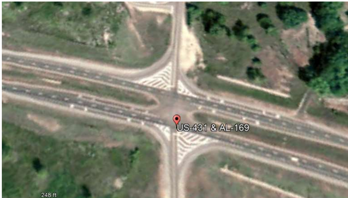
Figure 23. US 431 at SR 169 Before Condition (Google Earth)
