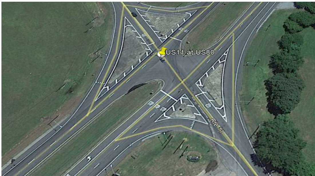
Figure 22. US 11 at US 80 After Condition (Google Earth)
