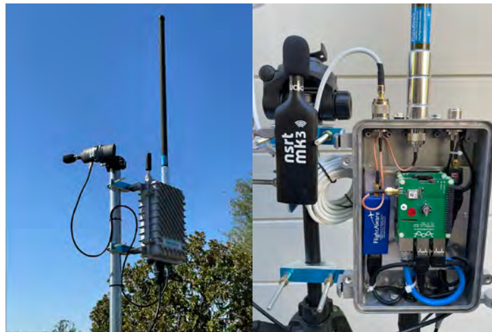
Figure 2. Sensor controller rooftop deployment with ADS-B and SLM (left); sensor controller components (right).
