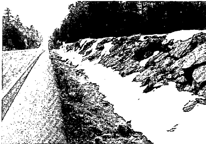
Figure 6. Rural roadside hazard rating of 6.
