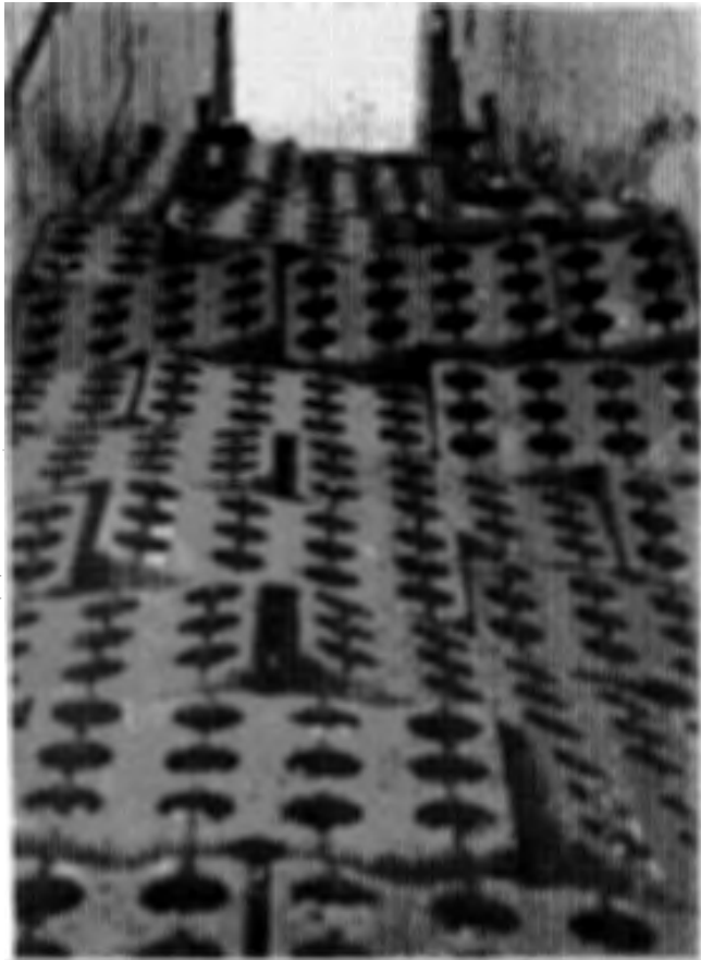
a. Looking downstream at the embankment shoulder.
