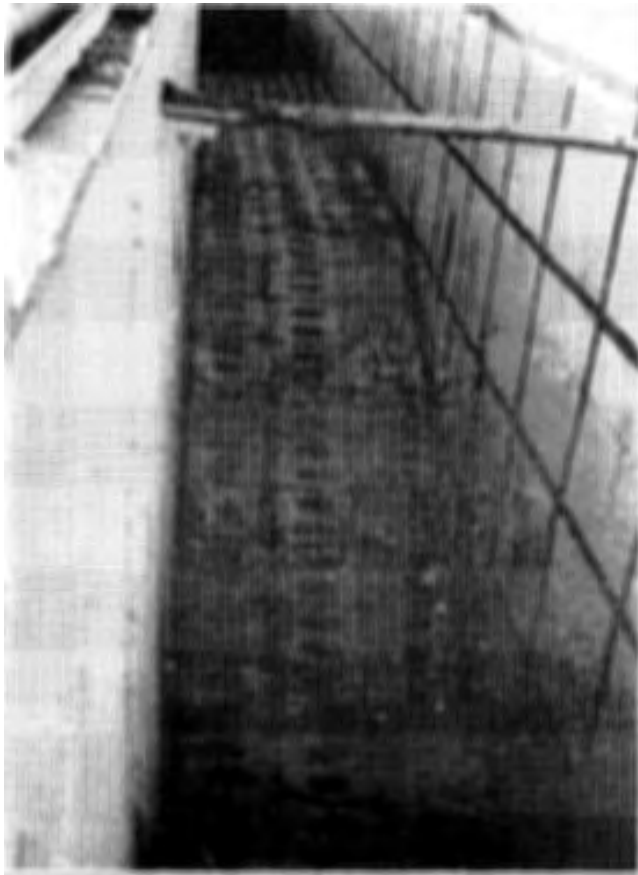
a. Looking upstream.
