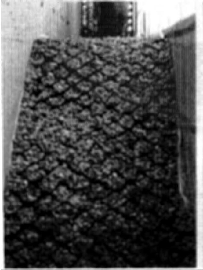
a. Looking upstream from the toe of the slope
