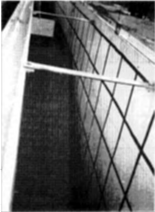
a. Looking upstream
