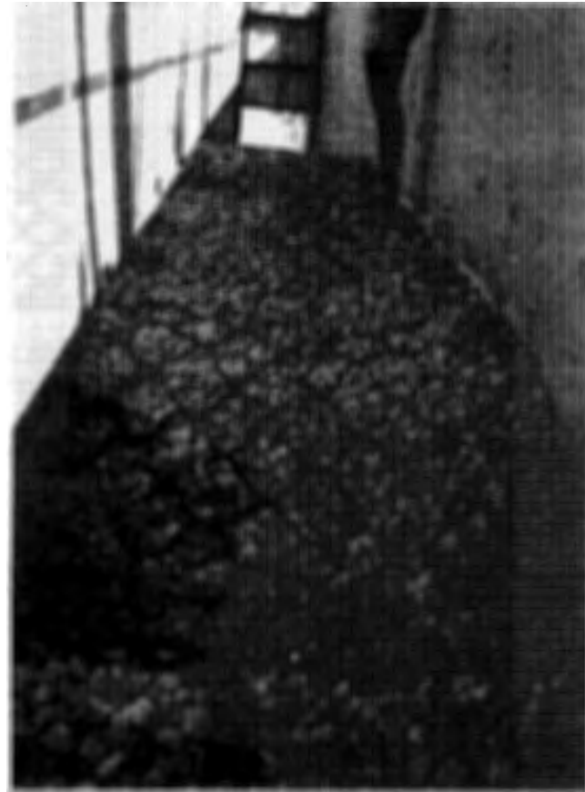
b. Looking downstream from the anchor trench.
