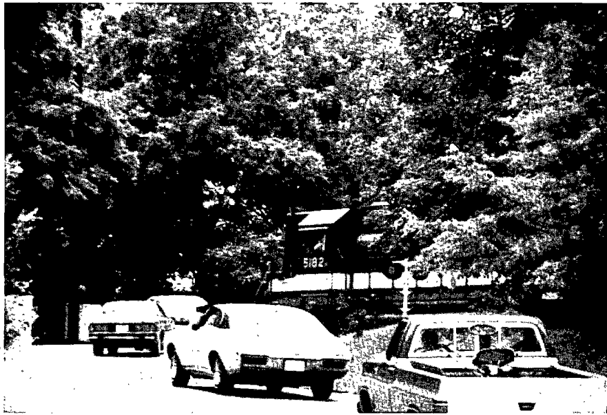
Figure 59. Crossing where sight distance to crossing is obscured.
