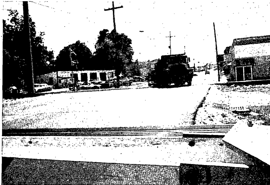
Figure 50. Tracks separated by sufficient distance to store motor vehicles.
