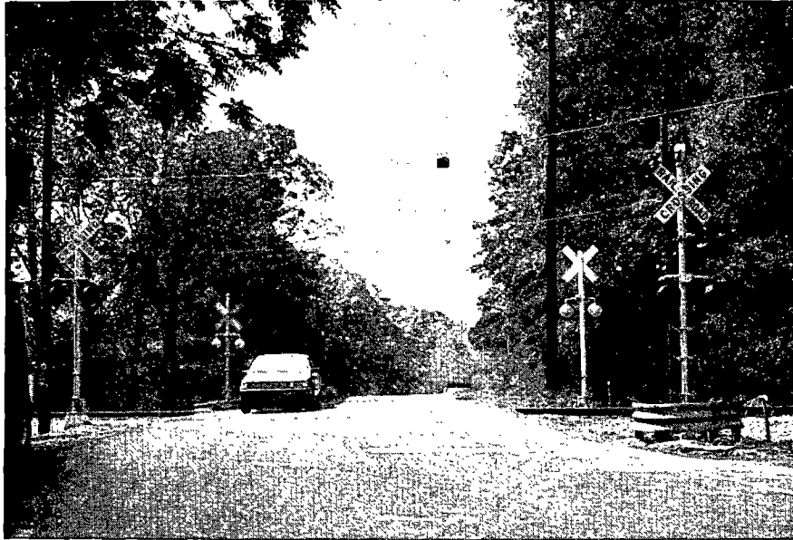
Figure 23. Four-quadrant flashing light signal system with overhead strobes installed at the Ebenezer Road crossing.
