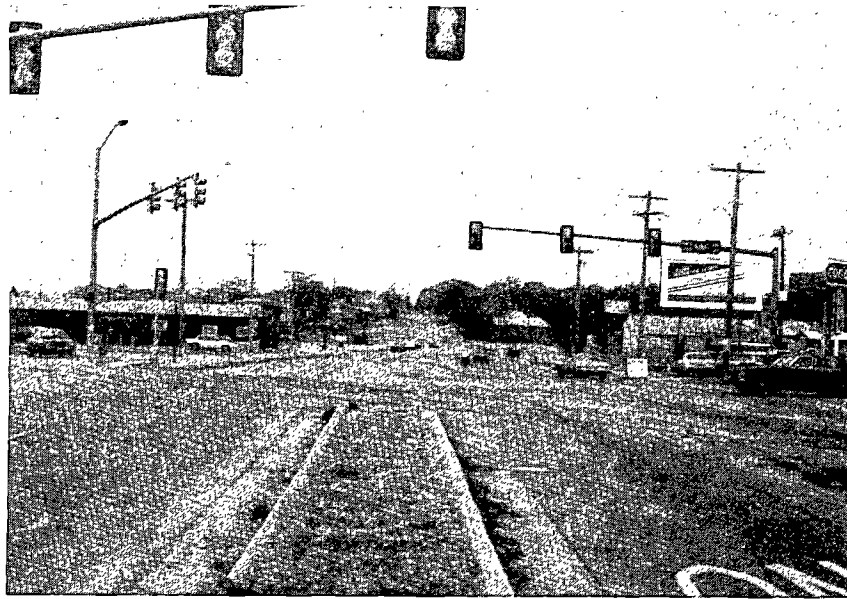
Figure 57. Highway traffic signals at crossing with complex roadway geometrics in Oklahoma City, Oklahoma.
