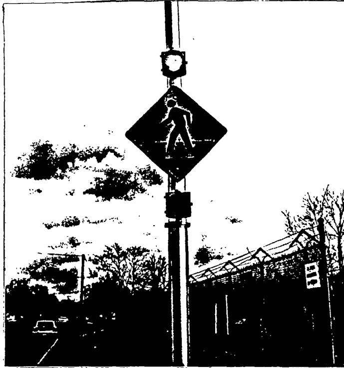
Figure 10. Pedestrian crossing sign and flashing signal.
