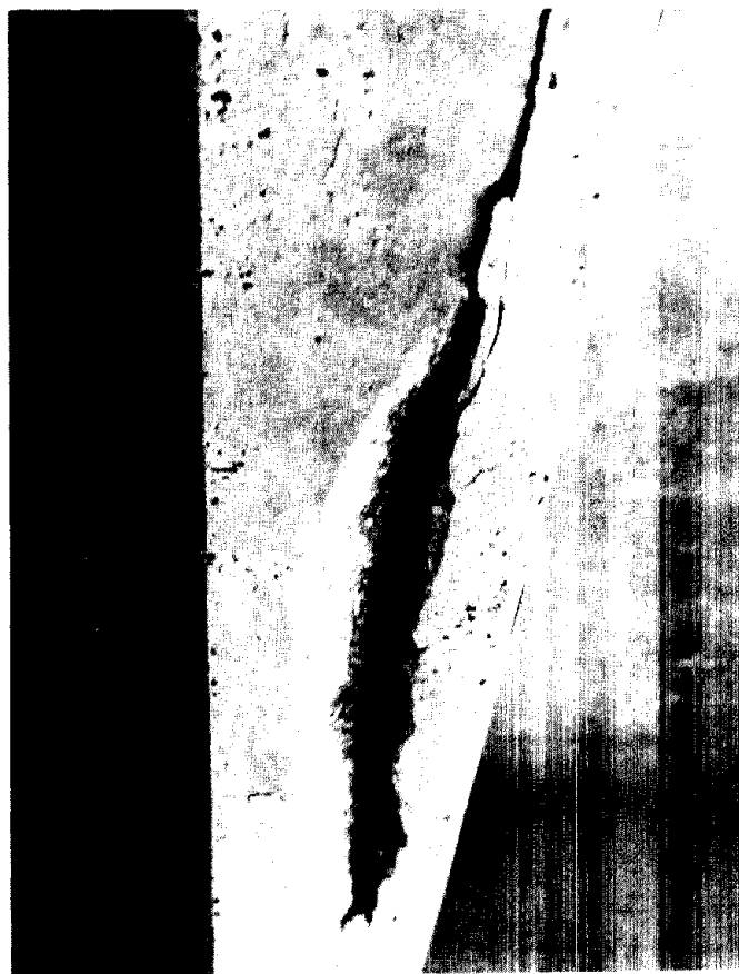
Figure 88. Spalling of concrete cover over the bottom tendon.
