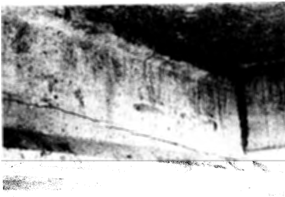
Figure 83. Cracking of concrete cover over a top tendon.
