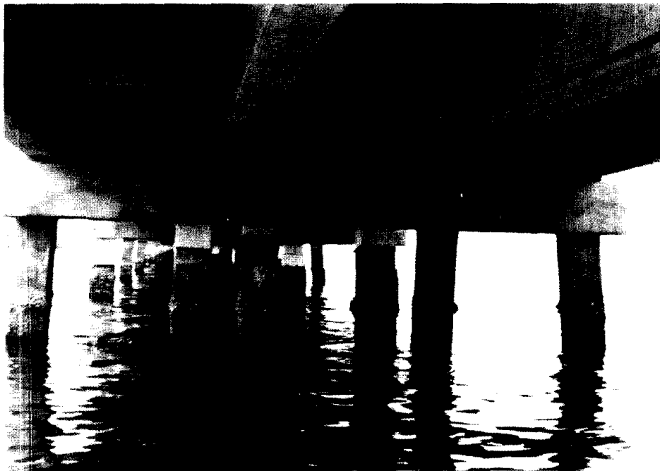
Figure 90. Remains of the protection system on prestressed piles.
