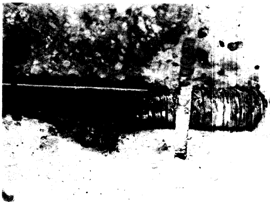
Figure 60. Condition of the newly exposed surfaces of the duct and the high chair rod in Girder 3.
