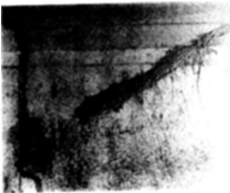
Figure 108. Crack repaired with an epoxy resin paste.
