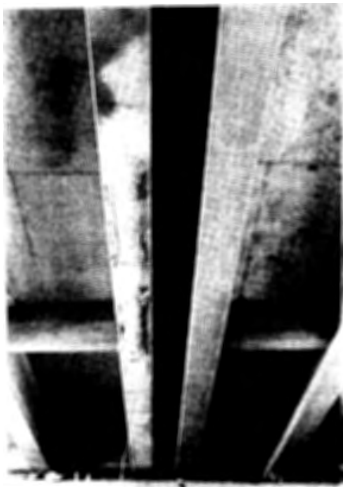
Figure 6. Spalling of concrete cover in Girder 3, Span 4.
