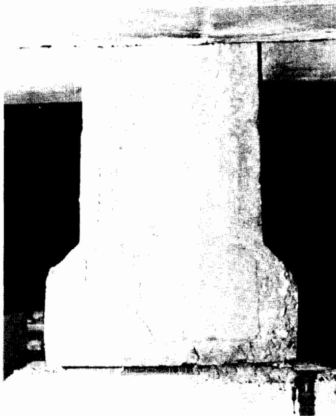
Figure 67. Cracks in mortar and concrete in areas of anchor plates.
