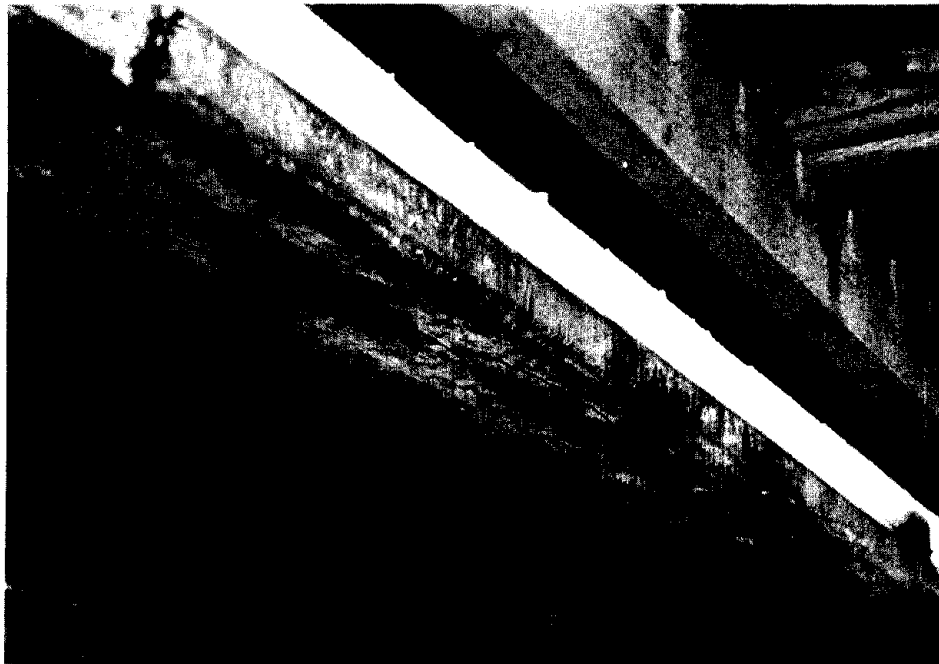
Figure 86. Rust stains around cracks in the bottom surface of a girder.
