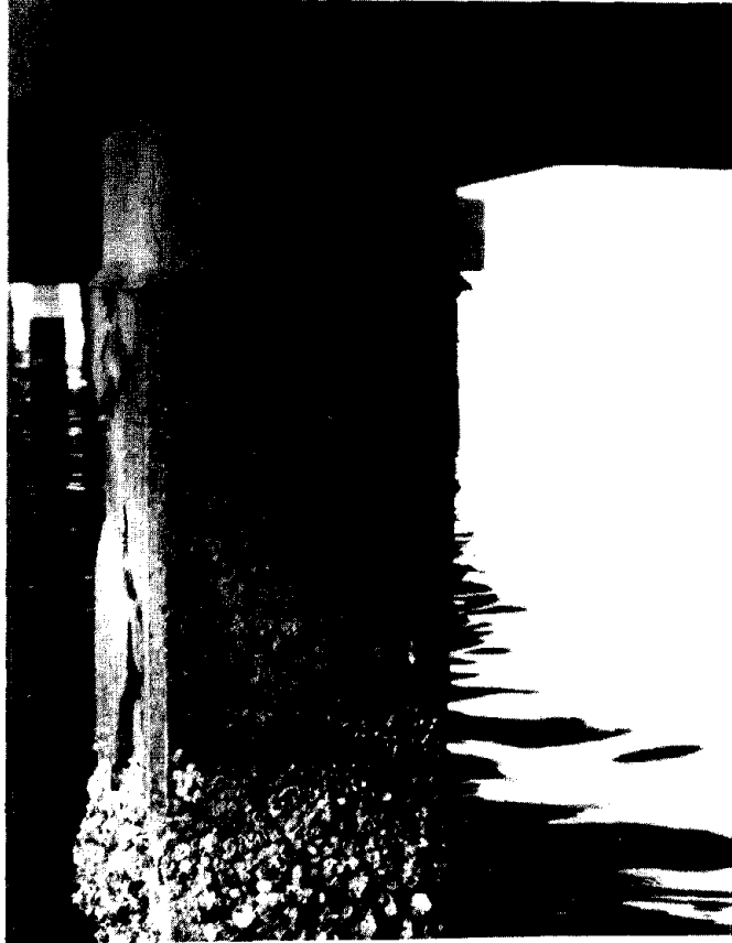
Figure 89. Typical cracks in a prestressed pile.
