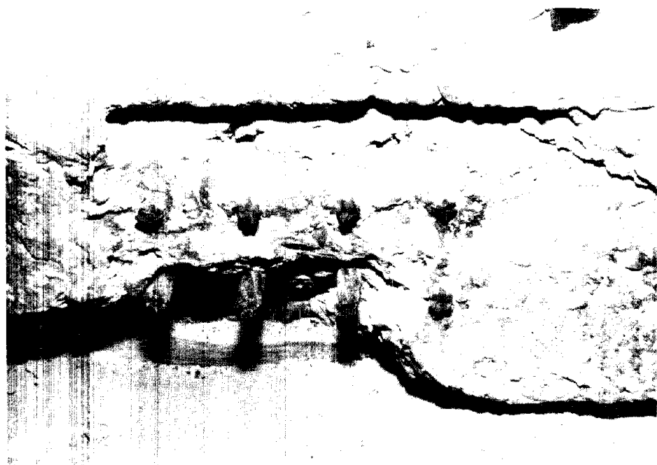
Figure 65. Moderate corrosion of exposed strands at the end of a girder.
