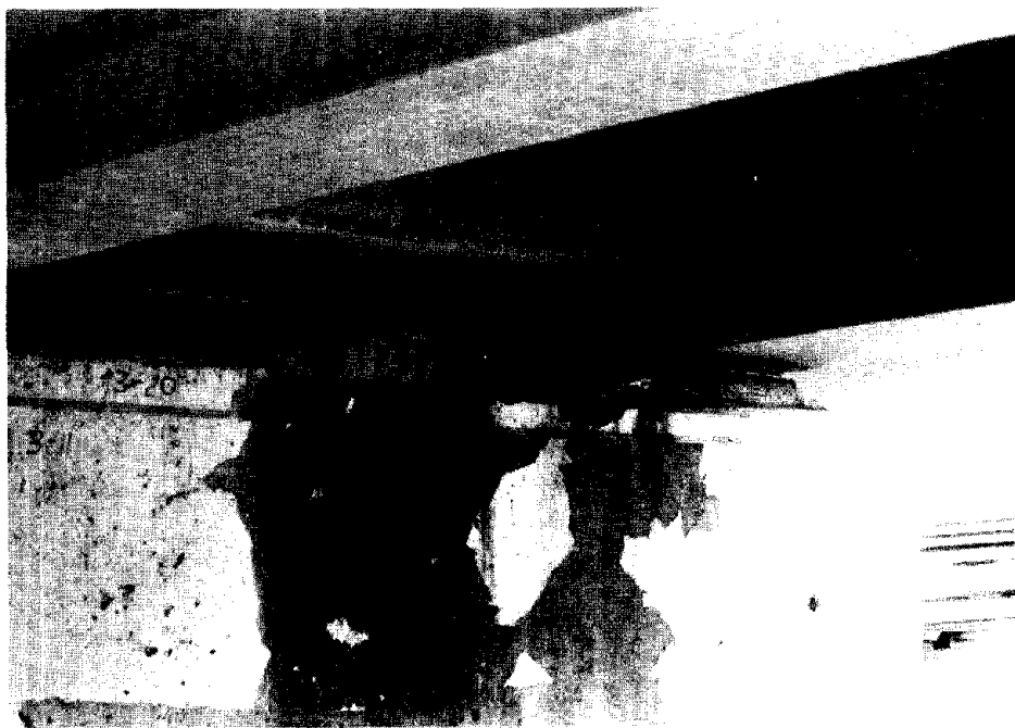
Figure 15. Cracking and spalling of concrete cover in diaphragms adjacent to transverse leaking joints.
