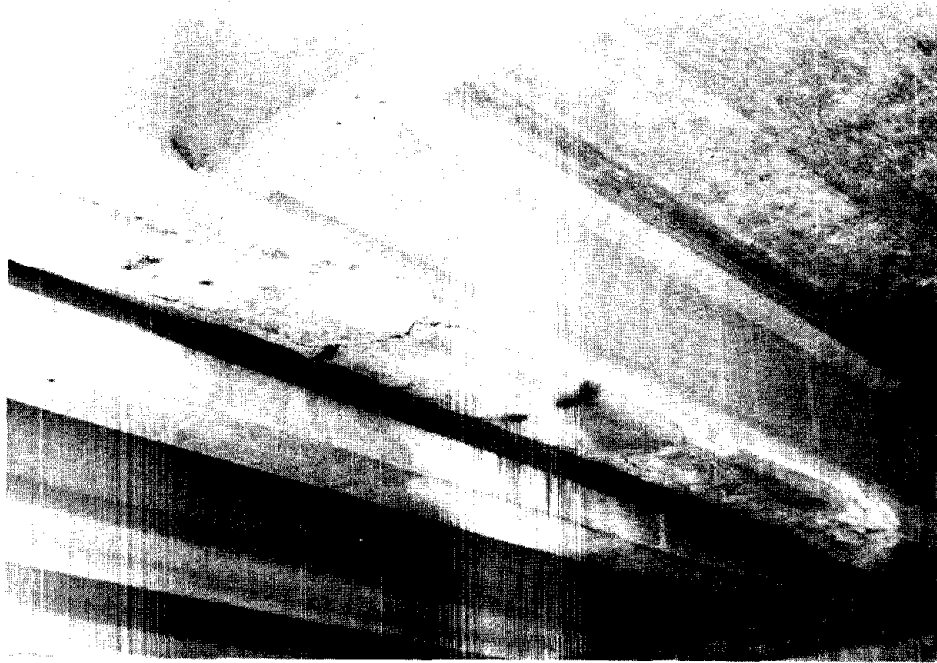
Figure 14. Cracks and stains of rust in the shotcrete patch.
