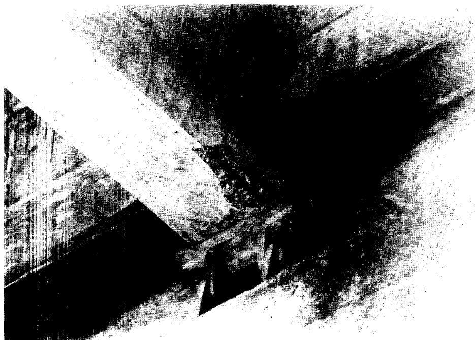
Figure 118. Spalling of concrete cover over conventional reinforcing steel bars.
