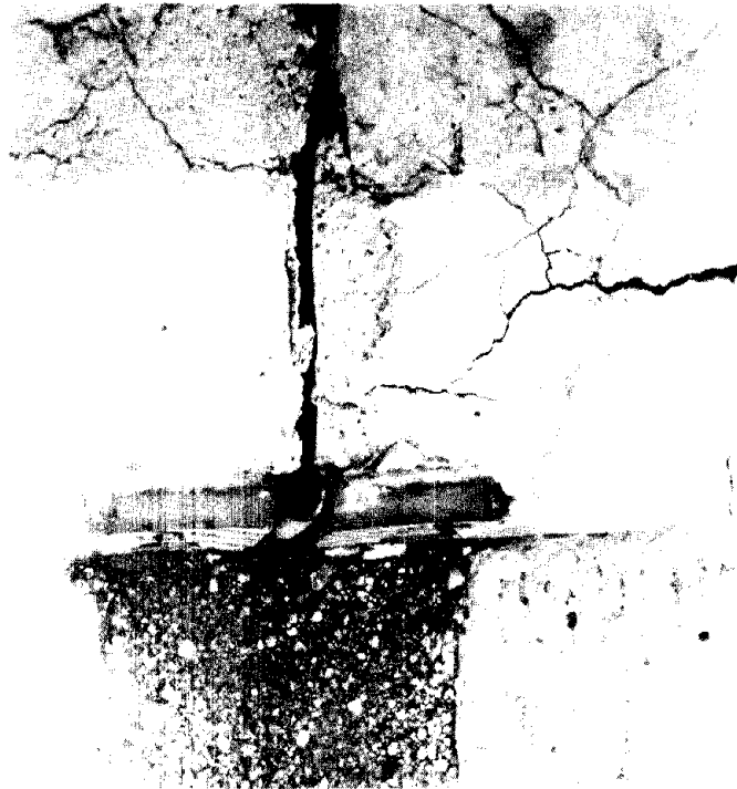
Figure 73. Accumulation of debris and deterioration of concrete in areas adjacent to the open sidewalk expansion joint.
