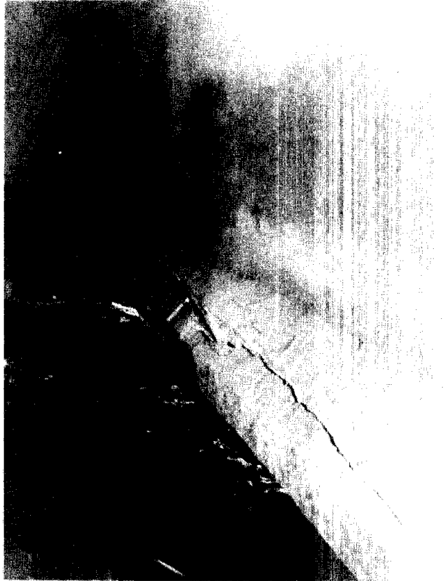
Figure 85. Cracking through the flange of a beam.
