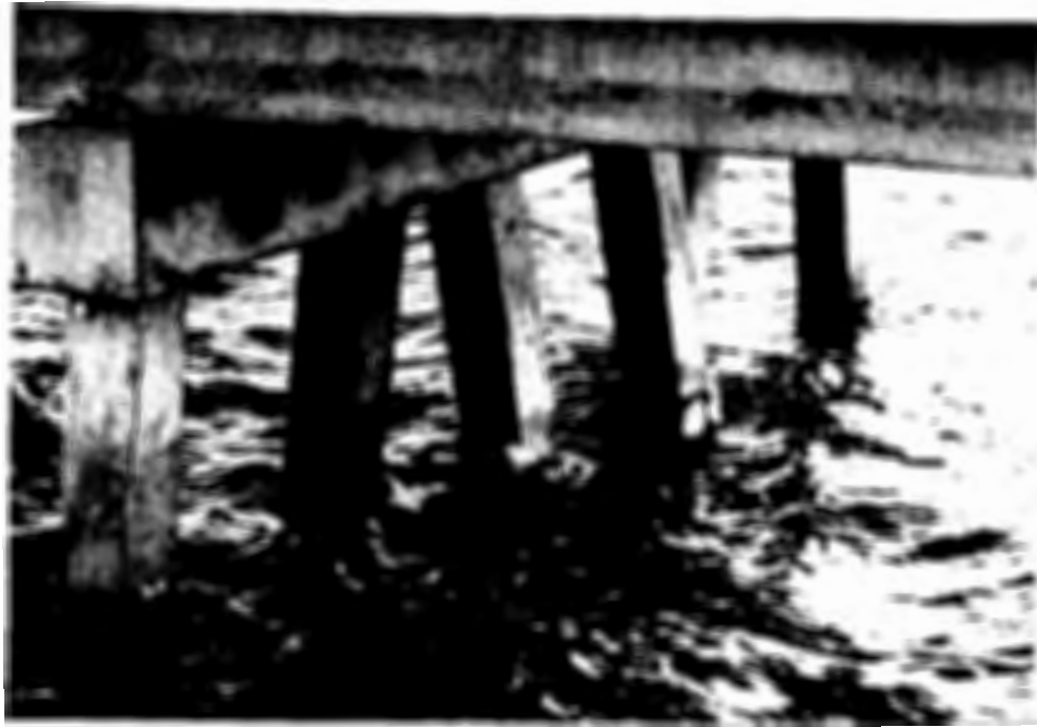
Figure 91. Cracks in prestressed piles of out-of-service Sunshine Skyway Bridge
