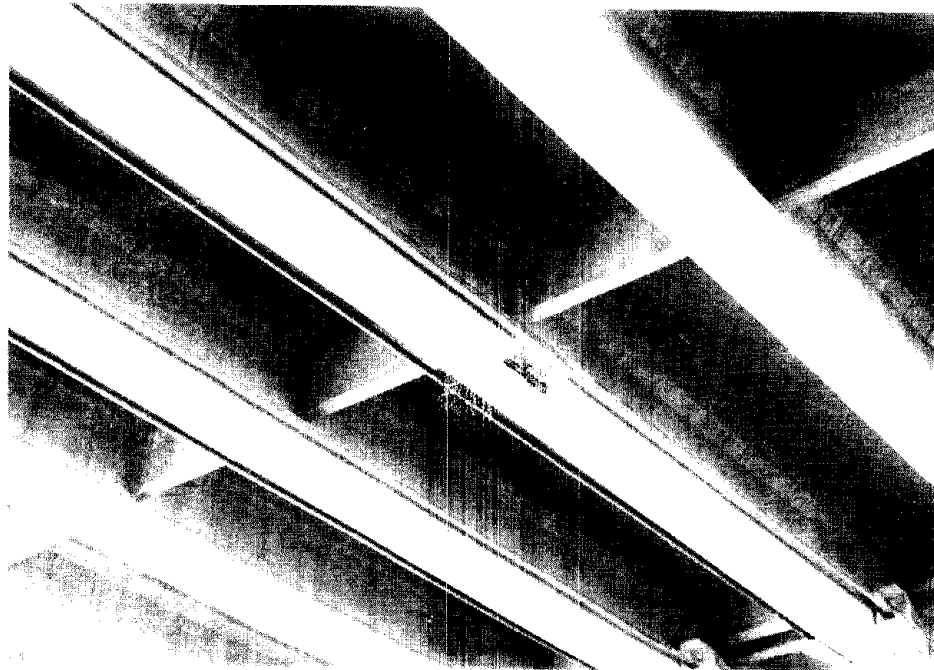
Figure 57. Exposed post-tensioned tendon in Girder 3, Span 36-37.
