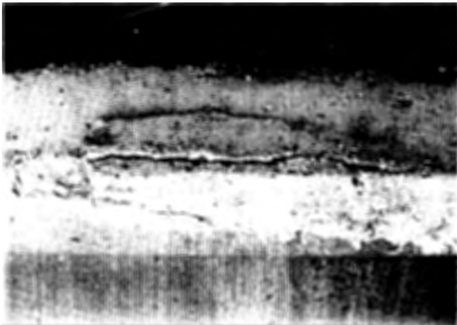
Figure 5. Severe cracking of concrete cover in Girder 3, Span 4.
