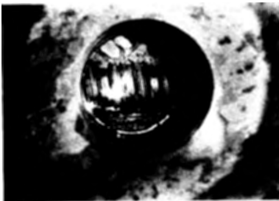
Figure 113. Exposed seven wire strand.
