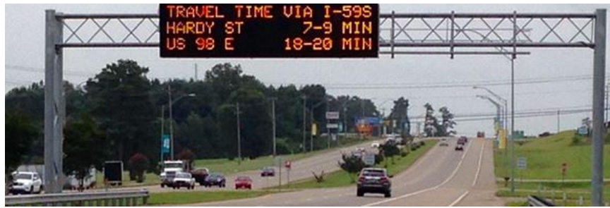
Figure 3.11. An example of a Dynamic Message Sign (DMS) showing estimated TT to nearby highway intersections.
