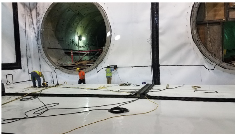
Figure 5-8 HDPE membrane installed in station area
