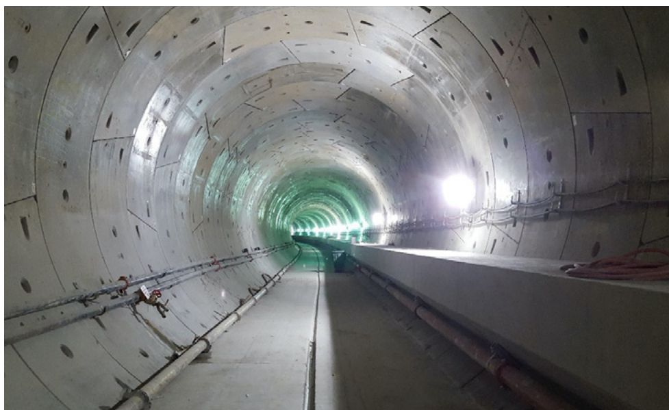
Figure 5-7 TBM tunnel (Courtesy of LA Metro)
