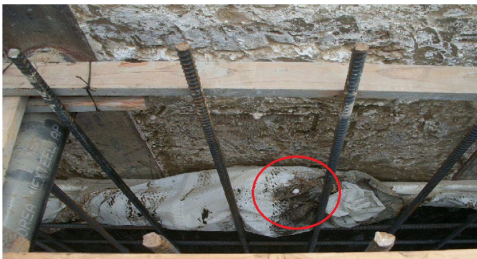
Figure 5-3 Nest in future concrete wall of WSX tunnel
