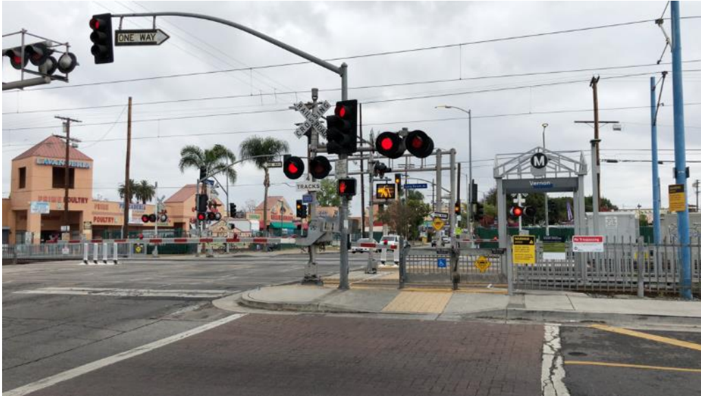
Figure 39: Signage and lighting
