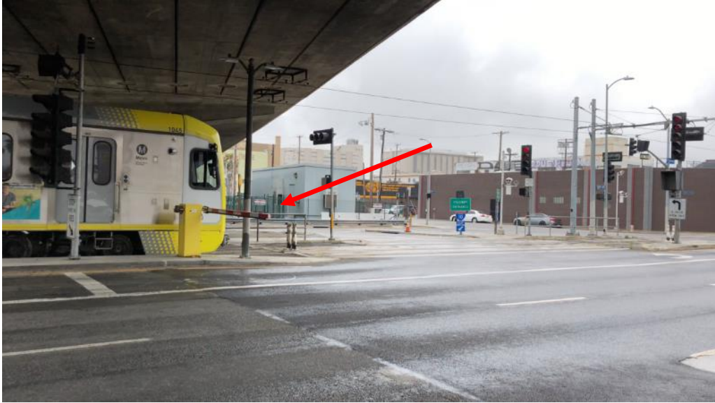
Figure 41: Parking lot-style gate
