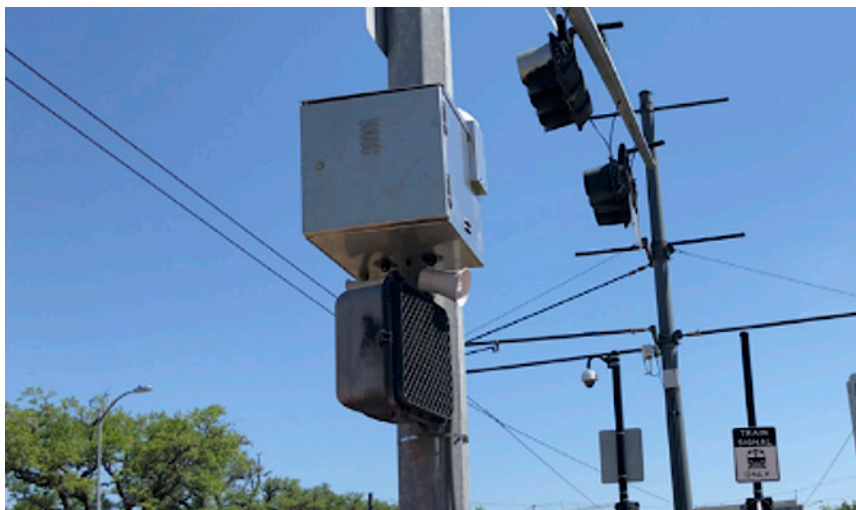
Figure 3-41 Bluetooth-enabled audio warning device
