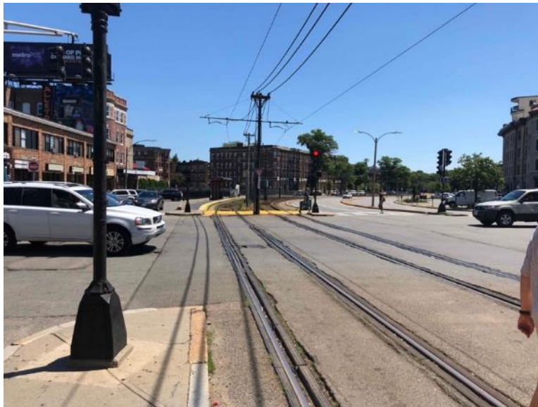
Figure 50: Typical level crossing
