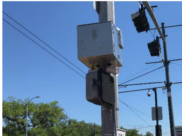
Figure 11: Bluetooth-enabled audio warning device
