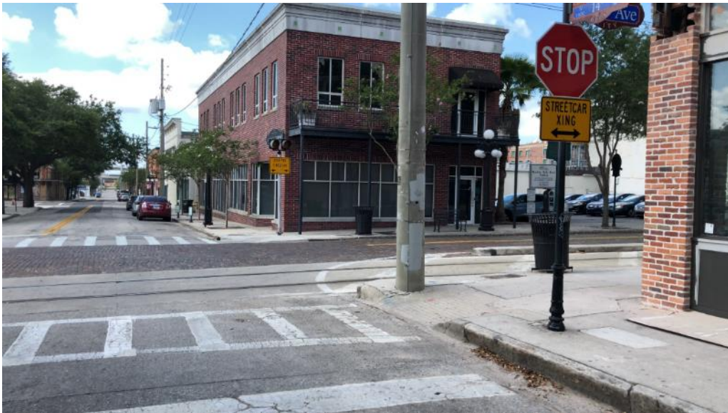
Figure 13: Poor line of sight from cross street
