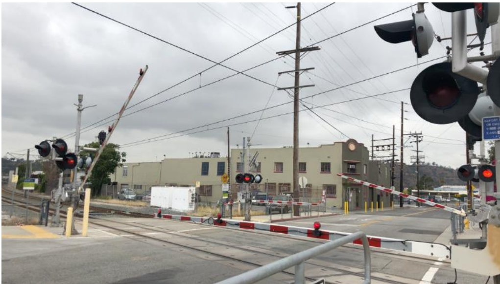
Figure 48: Four-quadrant gated crossing
