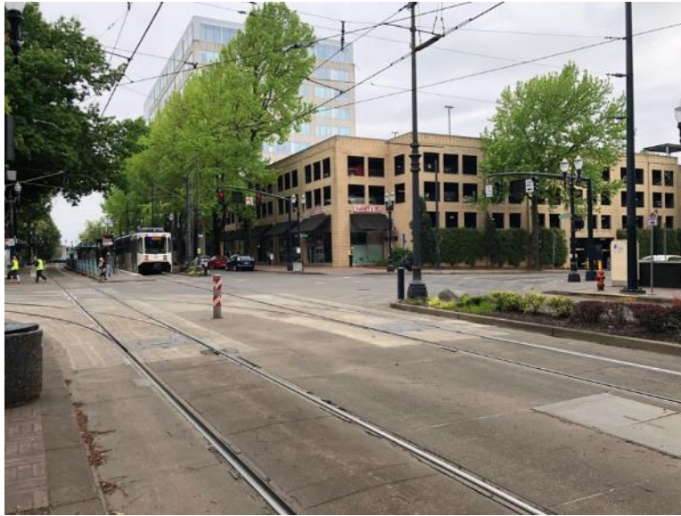
Figure 22: Holladay and 11th turning hazard
