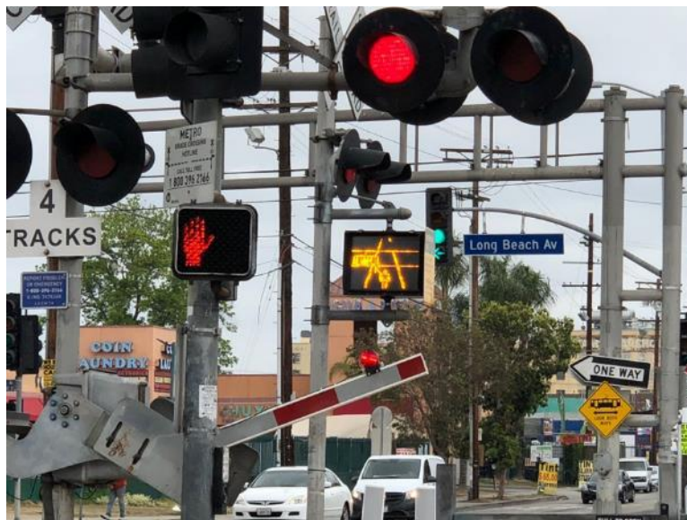
Figure 40: Signage and lighting
