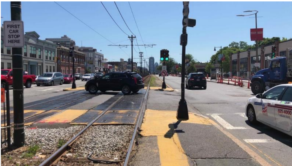
Figure 53: Illegal left turn
