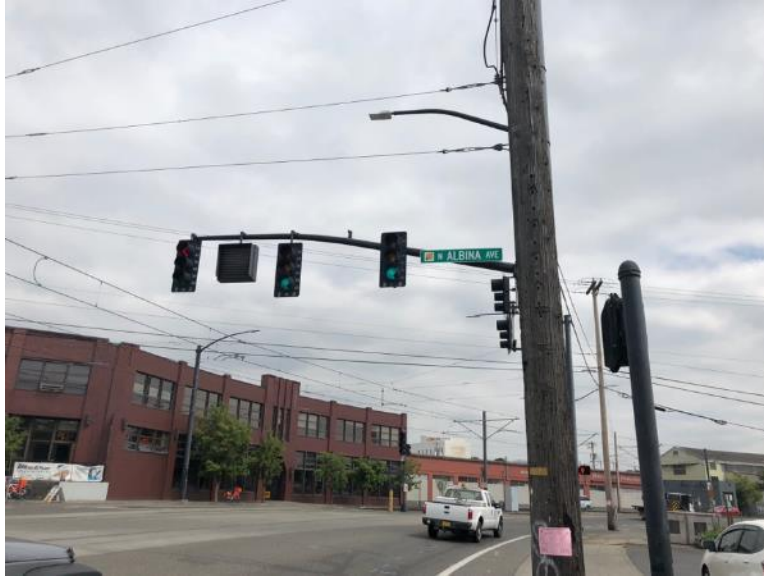
Figure 28: Signage and lighting
