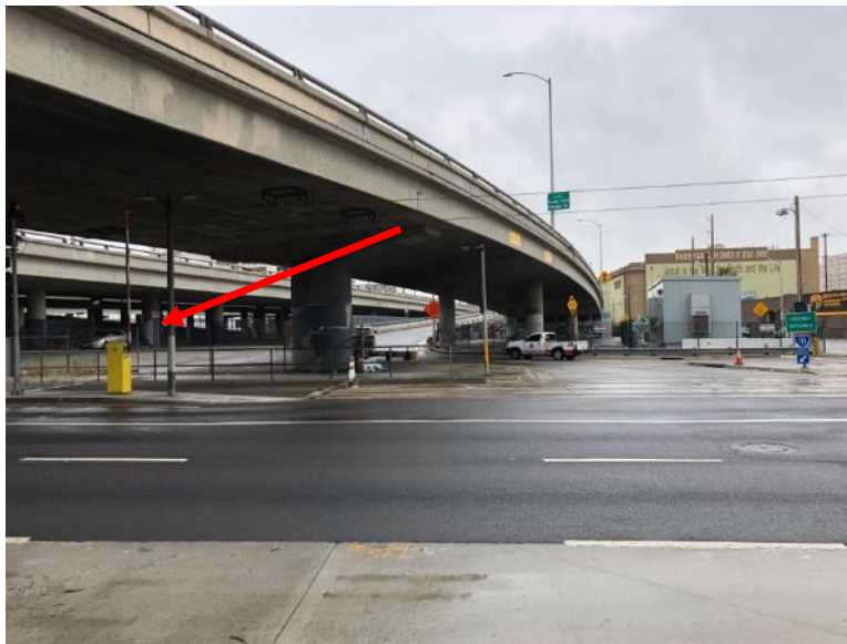
Figure 42: Parking lot-style gate
