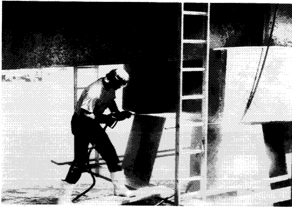
Figure 16. Cleaning of concrete surface prior to installation of zinc/hydrogel.
