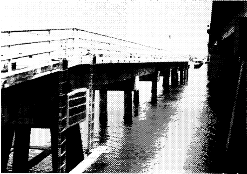
Figure 17. Zinc/hydrogel installed on bent #2 pile cap prior to painting.
