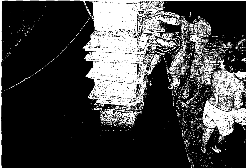
Figure 9. Pumping grout into installed pile jacket with horizontal bracing to prevent jacket deflection.
