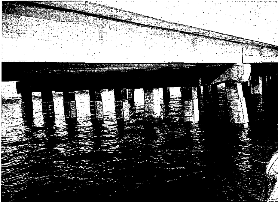
Figure 17. Bent with installed conductive rubber anodes.
