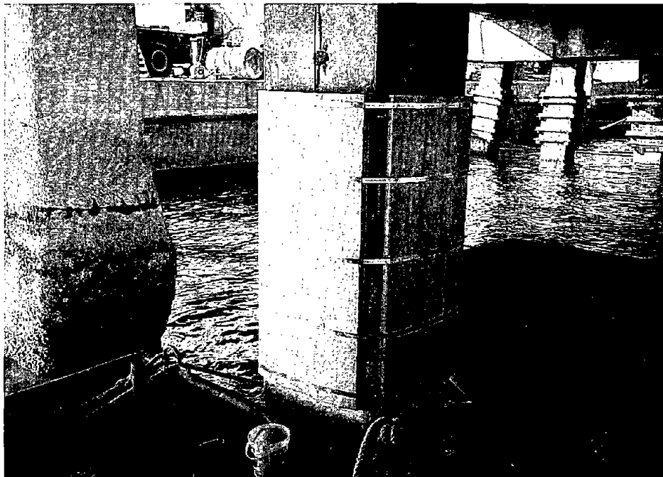
Figure 16. Installed conductive rubber anode.
