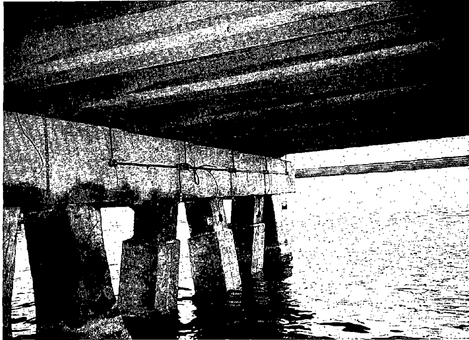
Figure 4. Wiring installation of zinc anode zone.
