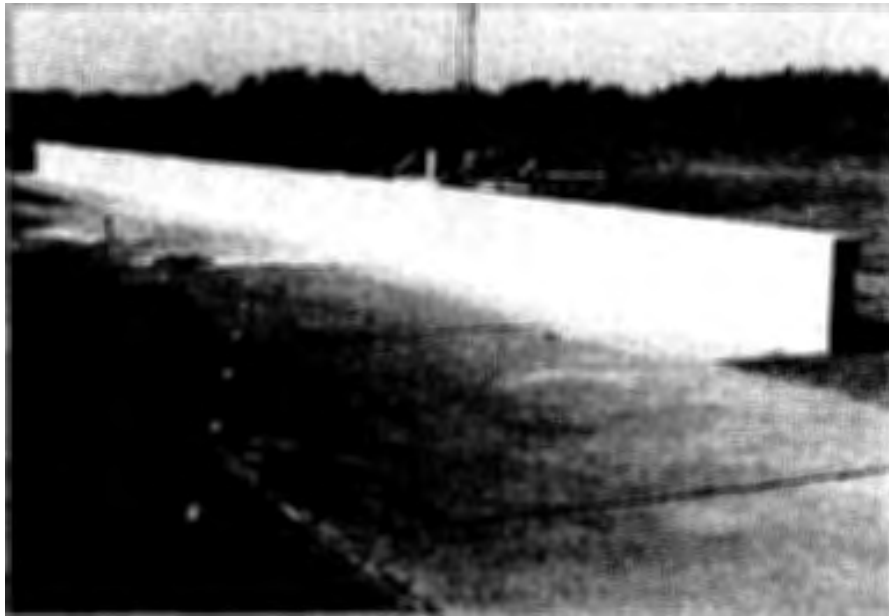
Figure 2. 32-in (813-mm) concrete parapet before test 7069-5.
