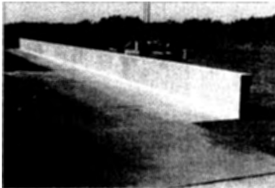
Figure 15. 32-in (813-mm) concrete parapet before test 7069-6.
