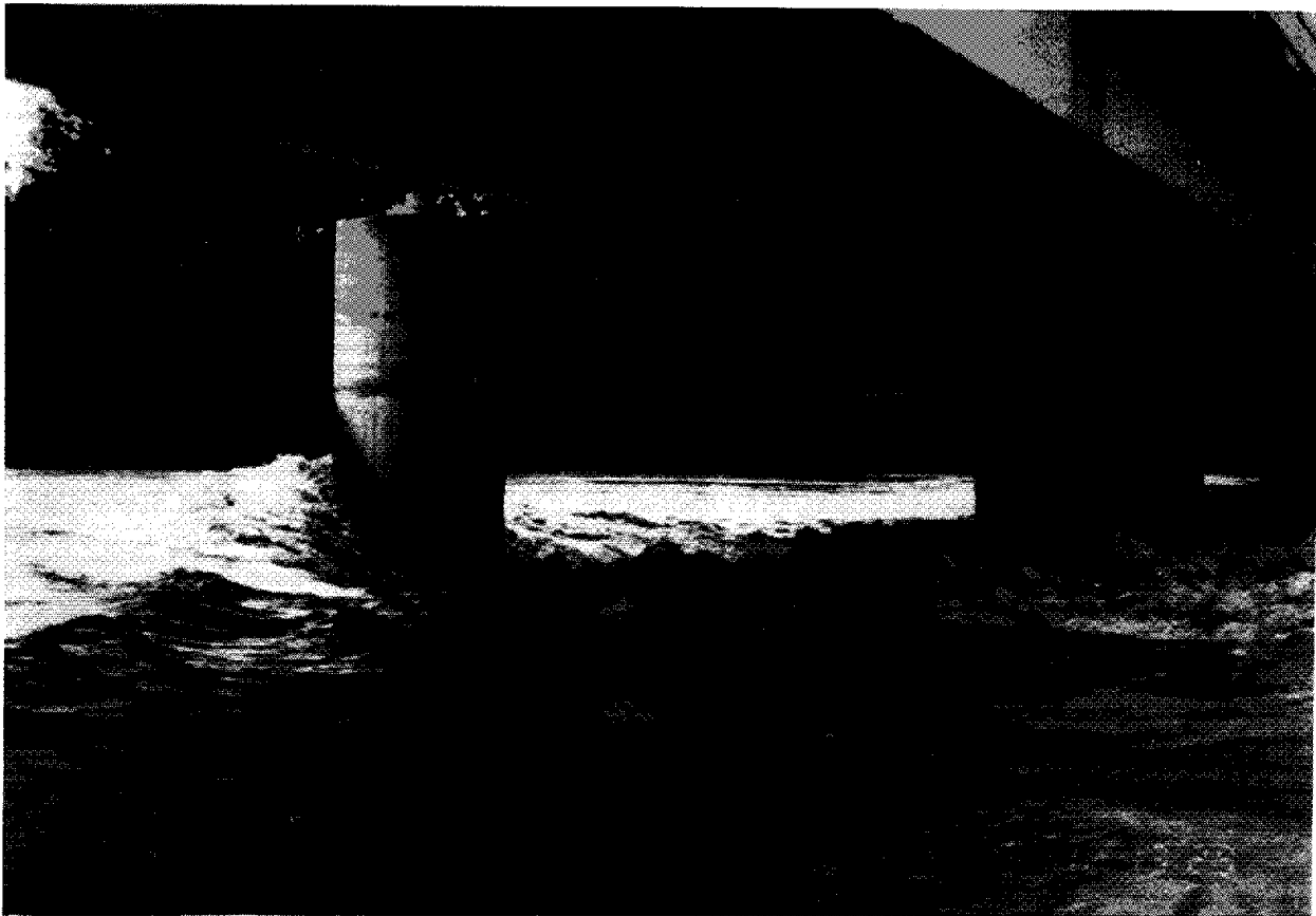
Figure 6. Bow wave and separation vortices at the nose of a pier.
