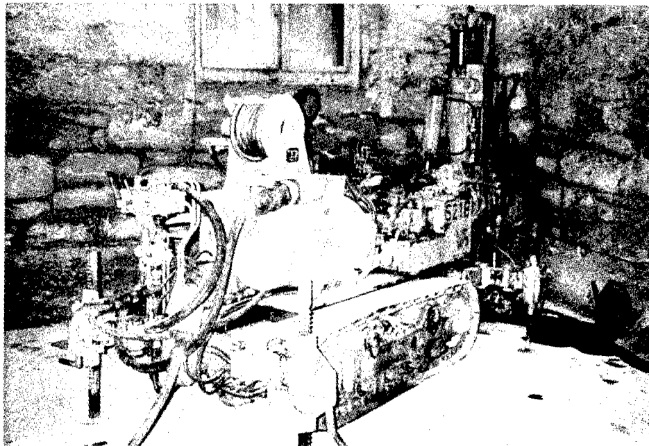
Figure 4. Similar micropile rig drilling in close proximity to wall. (Photograph courtesy of Hutte and Co.)
