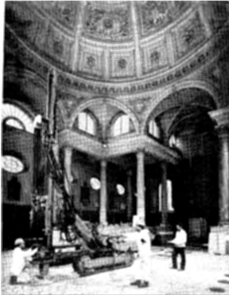
Figure 6. Example of contemporary diesel-hydraulic or electro-hydraulic track rig used for micropiling.
