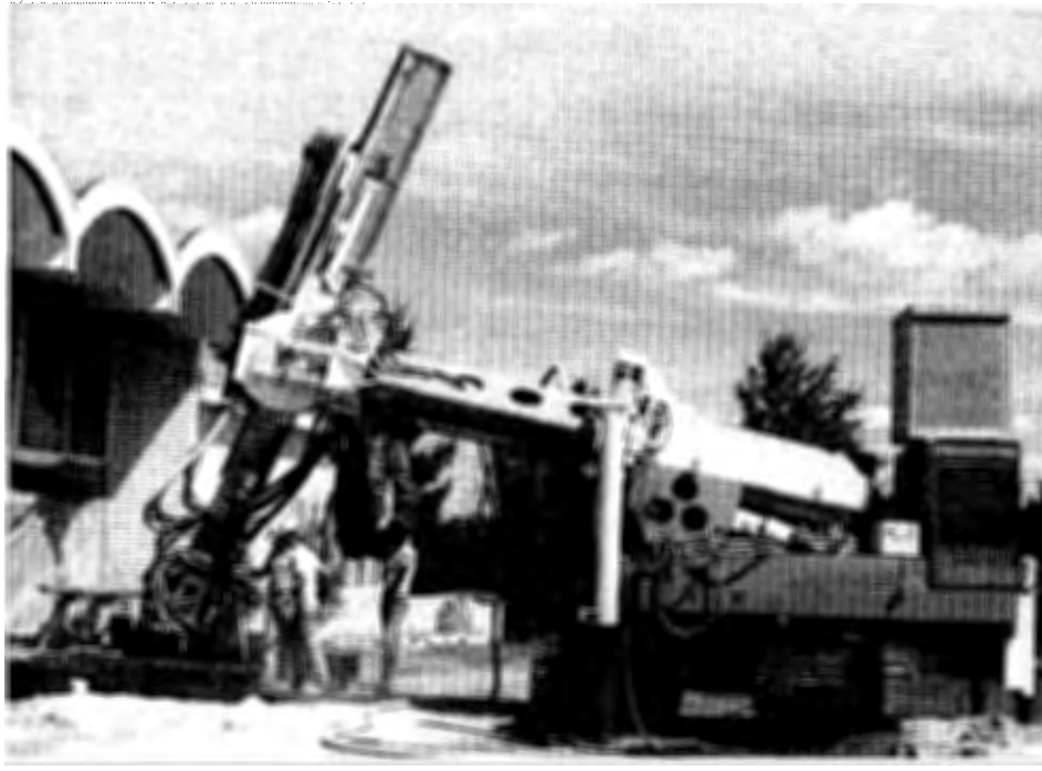
Figure 7. Diesel-hydraulic track rig drilling inclined micropiles.
