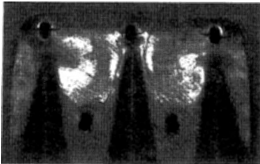
Figure 20. Interior damage to flat section, sample five.
