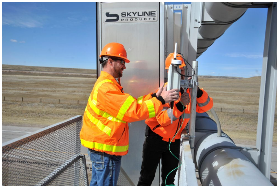
Figure 19. Wyoming RSU Installation along I-80.
