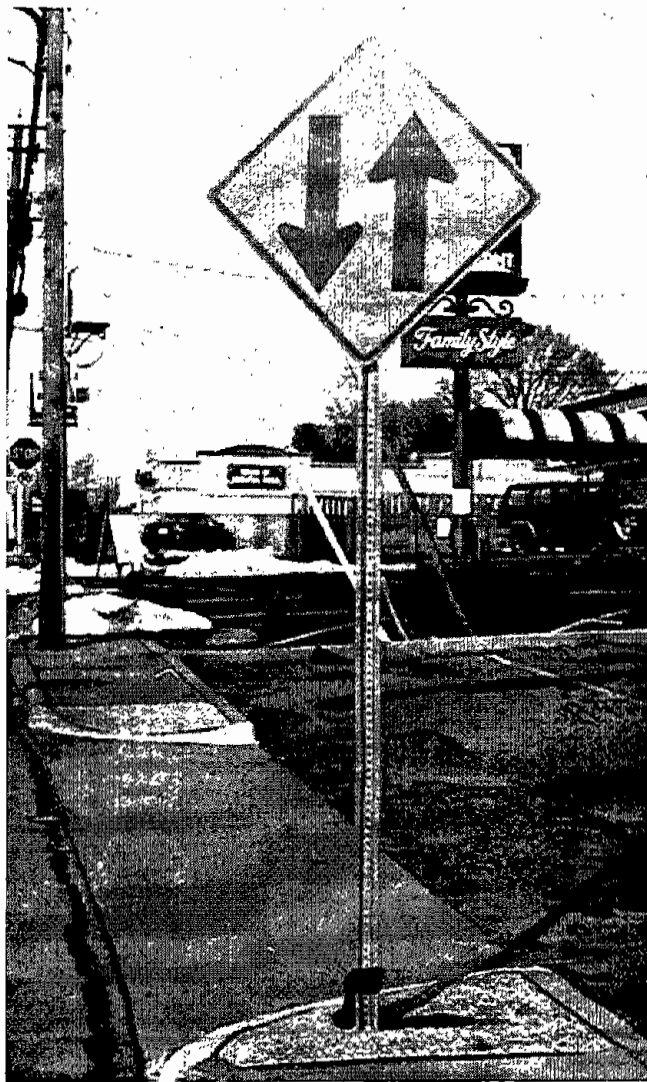
Figure 27 A flanged channel sign-support.
