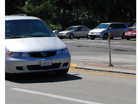
Despite a lane divider and delineator, drivers can misjudge a left turn on an arterial, resulting in wrong-way driving.
