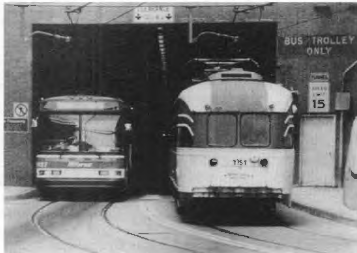
Figure 2. Bus and Electric Trolley Sharing Tunnel Right-of-Way
