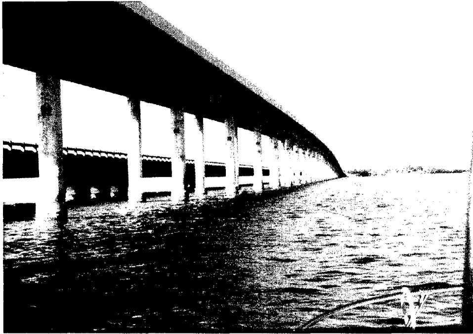
Figure 9. Niles Channel Bridge.
