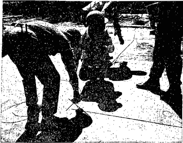
FIGURE 130.—Protective plates over sawed slots.
