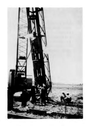
A5. it was natural that the engineer would turn to energy concepts, equating ram energy, Wh, to work done on the soil, Rs. Of course, rather gross assumptions were implied. The resistance of force, R, was assumed constant and the delivered energy was assumed to be the potential energy of the ram at the top of the stroke. The effects of cushions and helmets were neglected.
