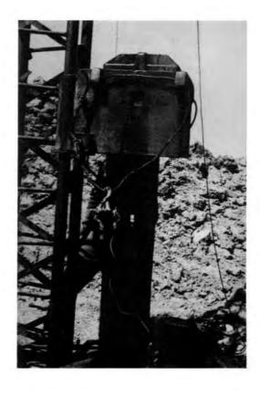
B45. For concrete piles a softwood cushion is placed between the helmet and the pile. The thickness of this cushion may vary widely.
