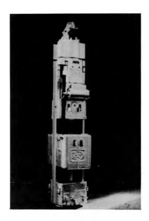
Bll. This slide shows another example of the double acting hammer. This particular machine operates on hydraulic fluid supplied by a pump. The system is a closed one since the spent fluid is returned to the pump. The pump is equipped to allow the control of the fluid pressure.
