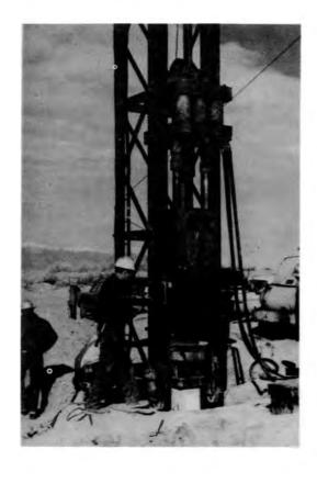
B12. The rating of both the single and double acting hammer assumes a predictable and constant energy. To include any energy losses the impact velocity is usually calculated using a reduced energy obtained by multiplication with an efficiency factor which is less than one. From the reduced energy an impact velocity can be calculated for input to the Wave Equation. Both hammer types can be handled in the same computer model.
