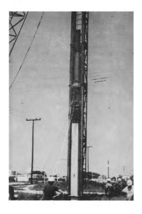
B21. In this photograph, another open end diesel hammer is shown. The impact block is partially extended and clearly visible at the bottom of the hammer.
