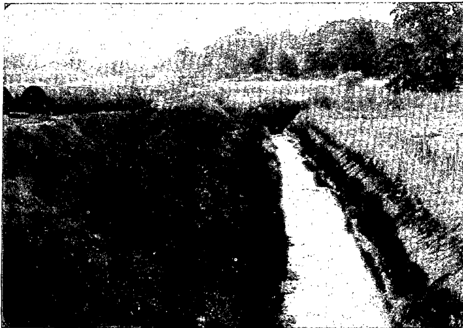
Figure 47. Sideslopes of fly ash embankment at Clophill By-pass prior to hydroseeding.
