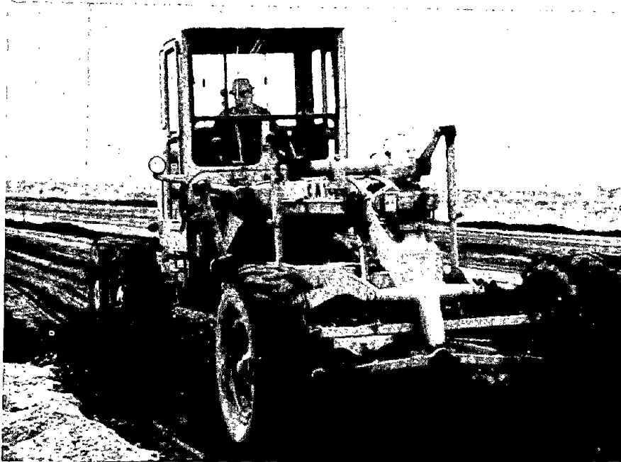
Figure 12. Spreading LCFA base course with motor patrol in confined areas at Newark Airport.
