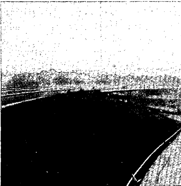
Figure 57. Construction of the M.23-M.25 interchange, England, where fly ash was used in the embankments and as structural backfill behind the bridge abutments.
