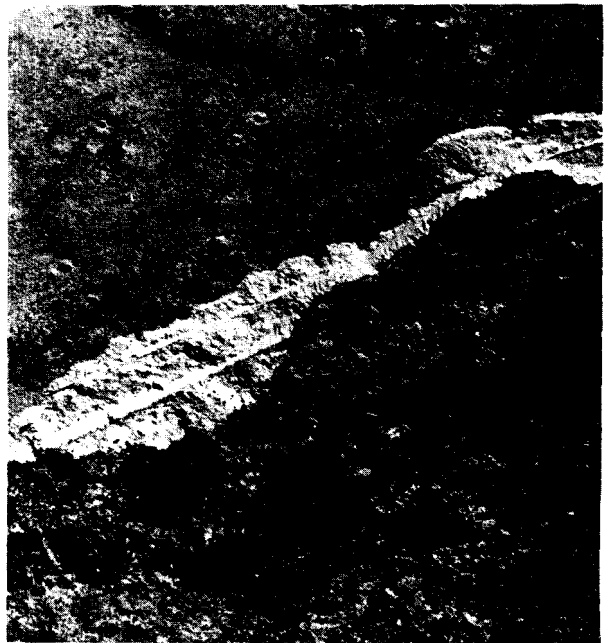
Figure 26. Close-up of Thermoplastic Removal by Special Grinding Tool
