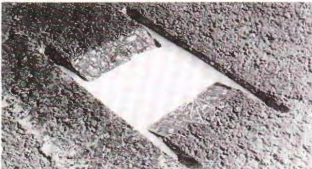
b) The sawed area is partially filled with an epoxy adhesive
