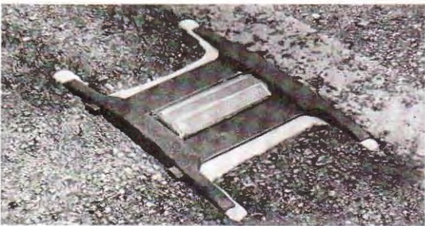
c) The Reflectorized Marker is placed into the pavement
