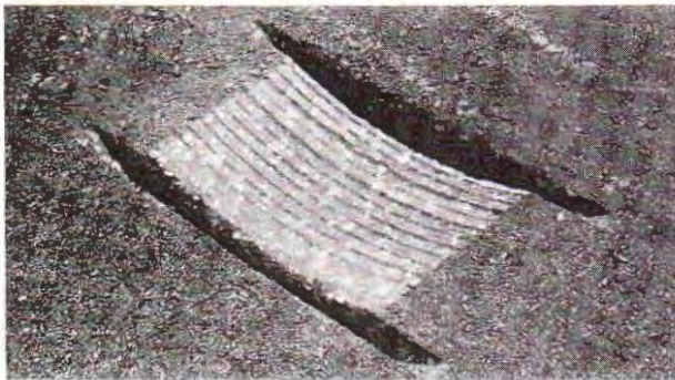
a) The pavement is cut to accept the marker
