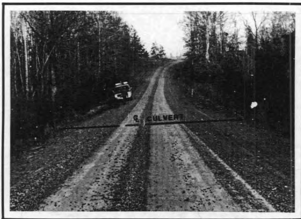
Exhibit 36. A line indicating a culvert centerline.
