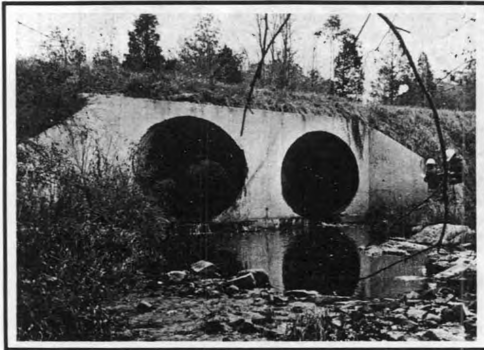
Exhibit 42. Headwall and wingwall end treatment.
