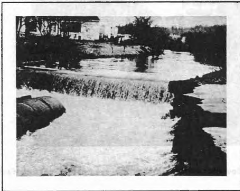
Exhibit 5. Roadway and embankment wash-out.
