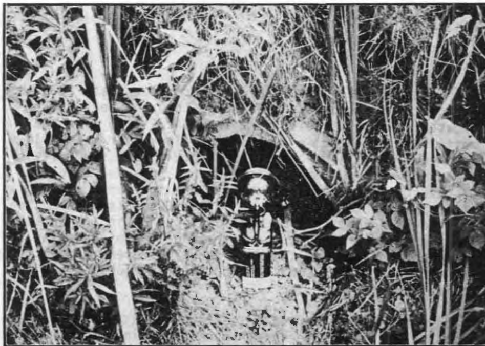
Exhibit 64. Culvert almost completely blocked by sediment accumulation.
