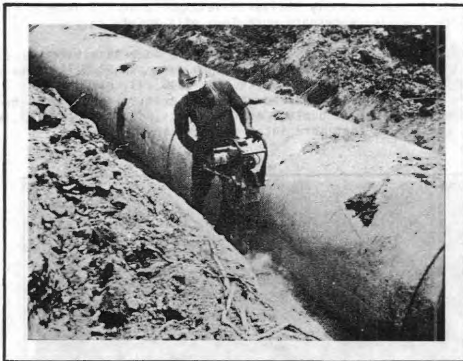
Exhibit 2. Attention to construction details such as compaction, bedding, and trench width is critical to proper culvert performance.
