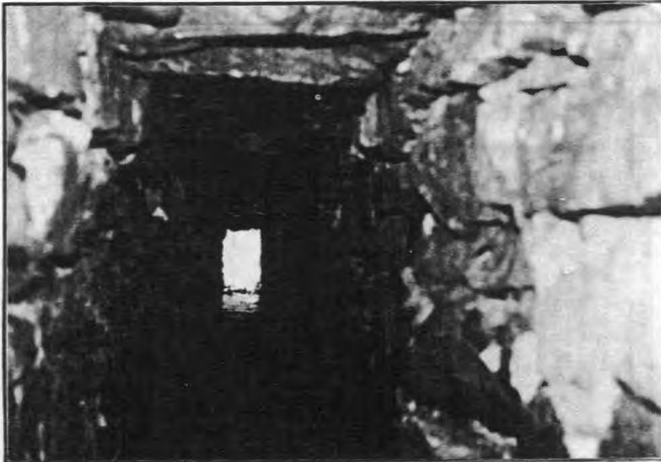
Exhibit 120. Dry masonry box culvert--rough worked stones without masonry.
