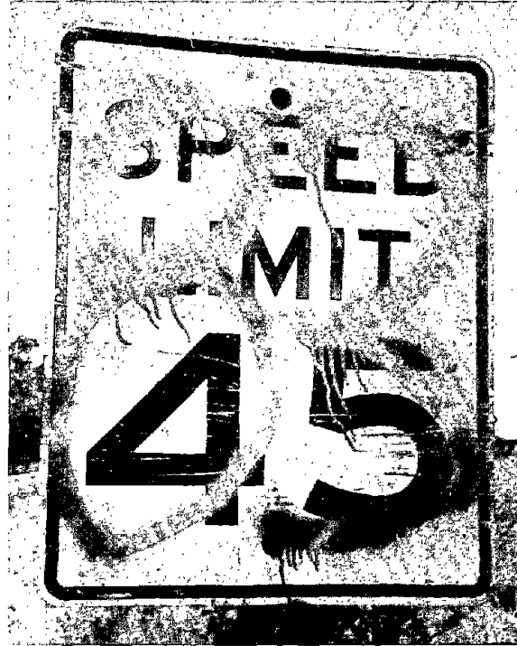
Figure 4. Example of mutilation due to spray paint.
