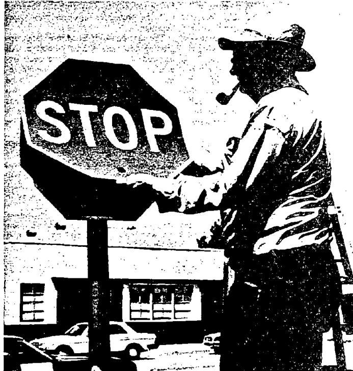
Maintenance Assistant Arnold Larsen overlays an El Monte stop sign with 3M high-intensity System 5 sheeting without removing the sign from the pole.
