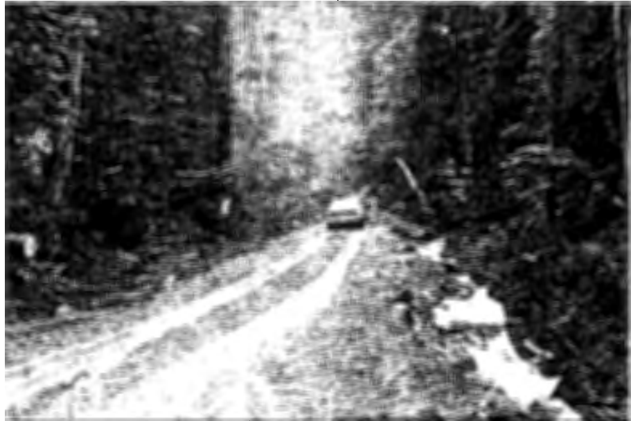
Figure 4-16: A completed road section adjacent to the clearing operation.
