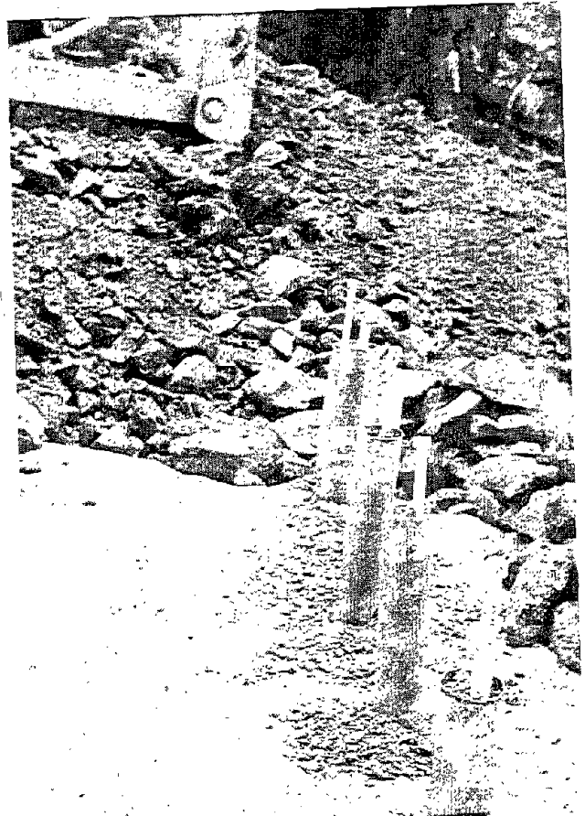
Figure 4-17: Settlement Plate Installation at Quinault.
