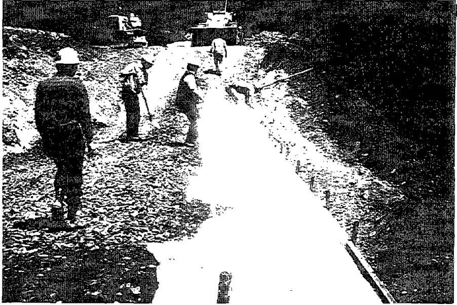
Overlap being made prior to placing next layer of fabric and backfill.
