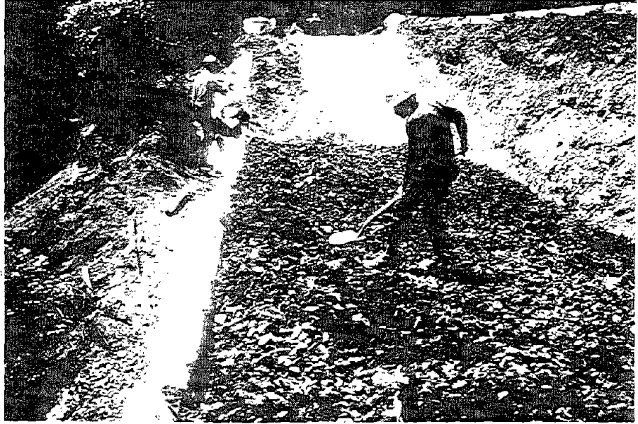
Backfill in place.
