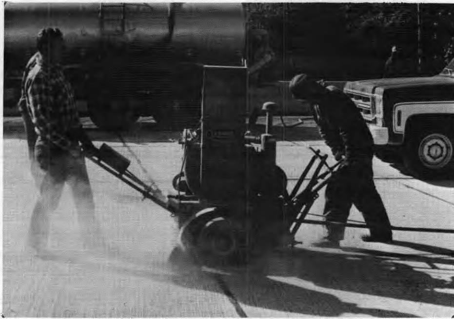
Figure 4. Tennant heavy-duty grinder (Model G). The operator of the machine could not keep true alignment; hence the laborer aided in guiding the machine.
