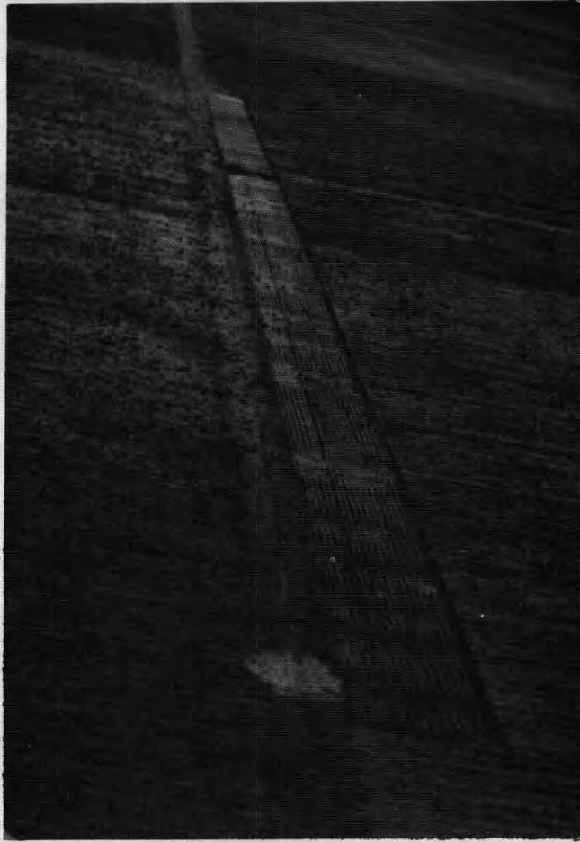
Figure 8. Recess formed by the Concut diamond saw. This method produced the truest vertical edges of the three methods used.
