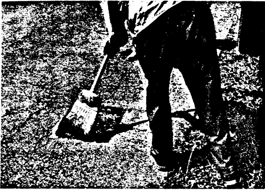
FIGURE 3.8 STEP 2. SWEEP CLEAN
