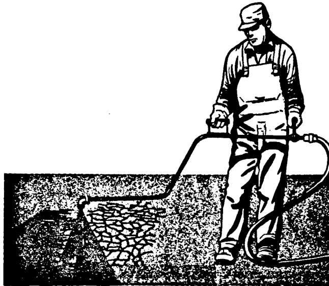
FIGURE 3.28 STEP 3. APPLY LIQUID ASPHALT
