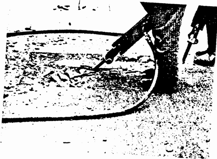
FIGURE 3.18 STEP 3. REMOVE UNSOUND CONCRETE
