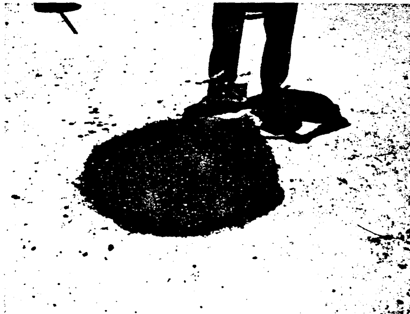
FIGURE 3.7 EMERGENCY PATCH WITH COLD MIX
