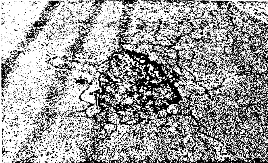
FIGURE 2.1 POTHOLES
