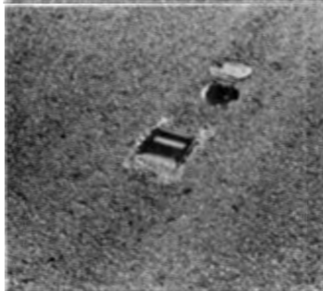
Figure A-6. Installation of Stimsonite 96 Marker.
