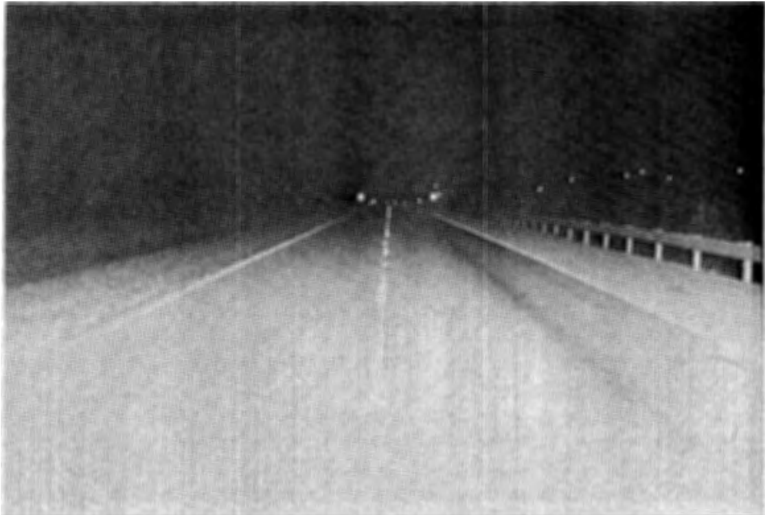
Figure 14. Photograph Taken at the Fayette County, Southbound Installation (Order of Markers is Kingray, Stimsonite 911, Stimsonite 96, Recessed, and Dura-Brite).
