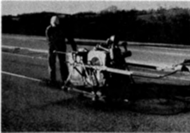
Sawing Groove
