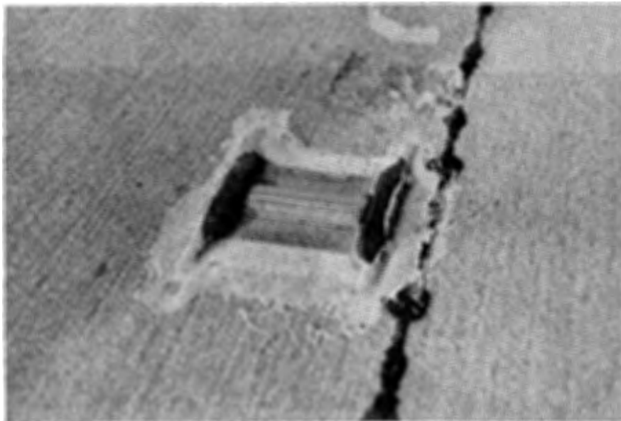
Figure 17. Stimsonite 96 Marker after Approximately One Year in Service (Before Snowplowing).
