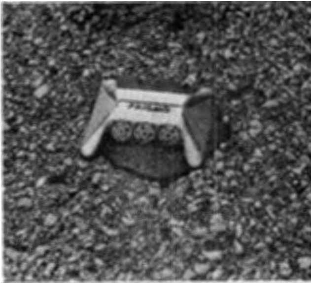
Figure 19. Prismo Marker after Approximately One Year in Service (Before Snowplowing).
