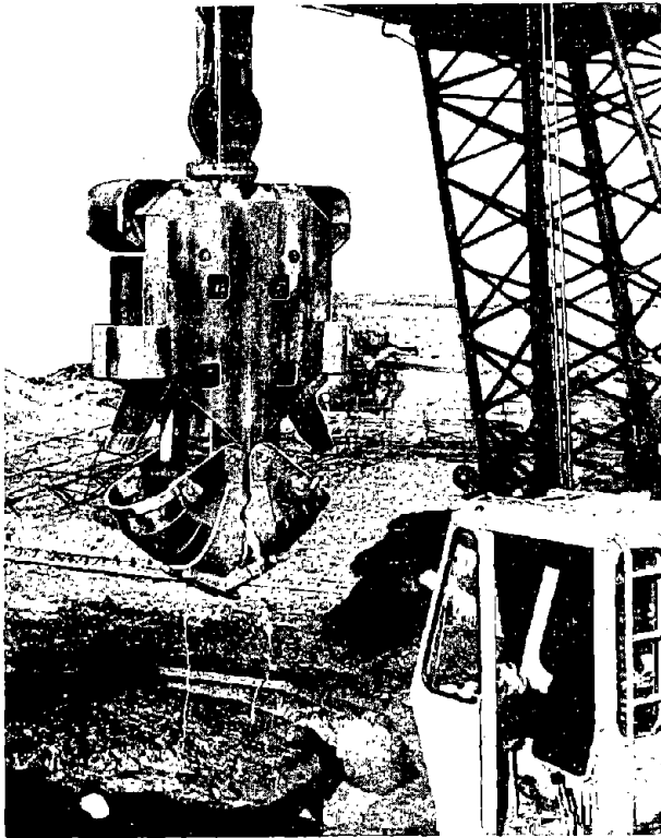
Fig. 10.3. -- Another type of grab bucket. Note overlapping of scoop teeth in closed position (Document from Gallia).
