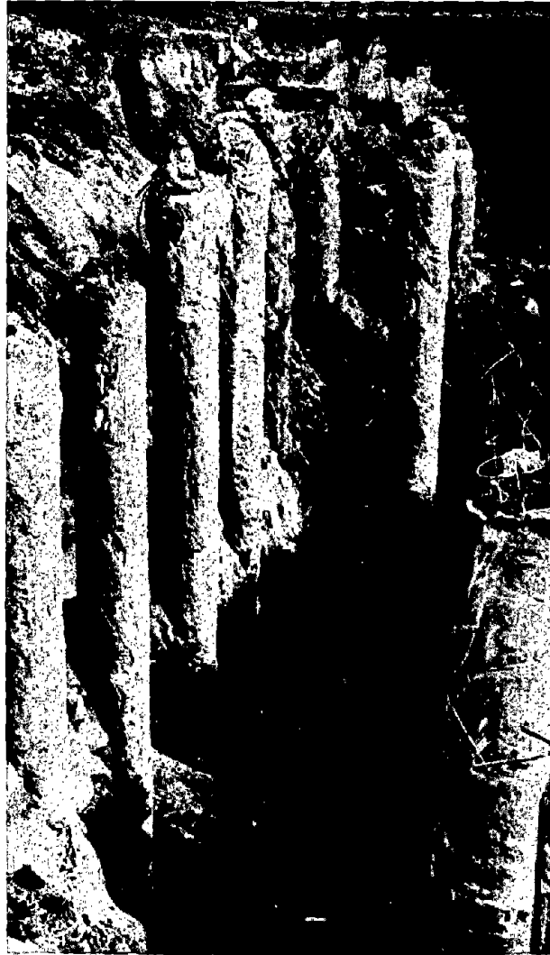
Fig. 151. -- Example of excessive trimming height.
