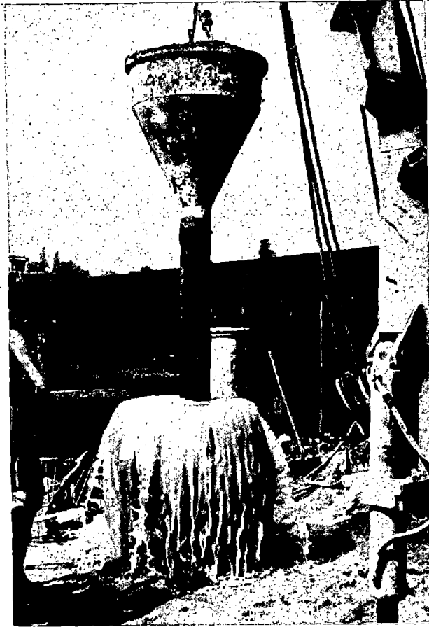
Fig. 126. -- Cone and pipe that form a tremie.
