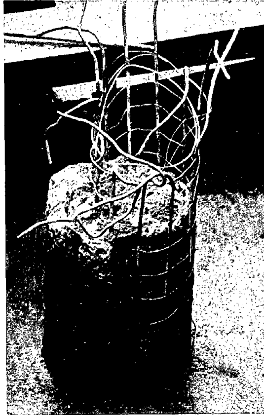
Fig. 183. -- Poor centering of reinforcing cage at head.
