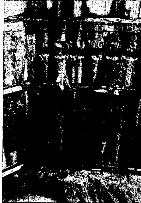
Fig. 40. -- Secant piles required because of significant water flow within a gravel layer.
