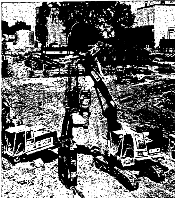
Fig. 10.5. -- Bucket suspended by derrick of hydraulic shovel (Document from Poclair).
