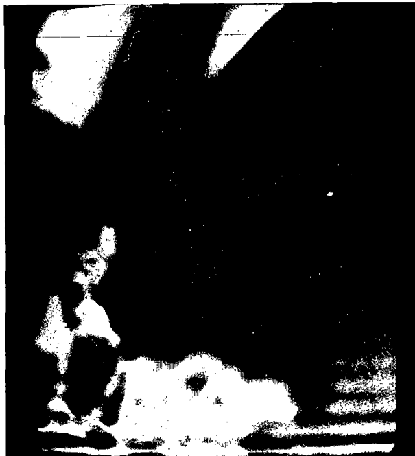
Fig. 167. -- Axial view: bottom of defective pile. Seen are a vertical rebar of reinforcing cage (on top) and a horizontal rebar of basket (below). The central black circle is lighting support.
