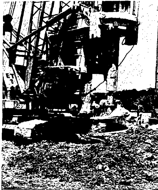
Fig. 9. -- Drilling of first meters.
