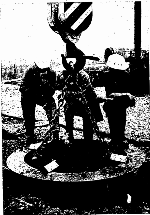
Fig. 70. -- Support at top of a casing with welded brackets.
