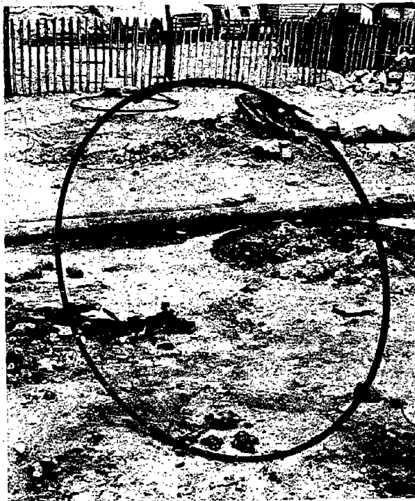
Fig. 86. -- Gauge hoop with overlapping welds with markings for position of longitudinal steel.
