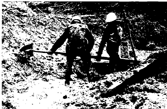
Fig. 12 and 13. -- Evacuation of debris at proper time. Required!
