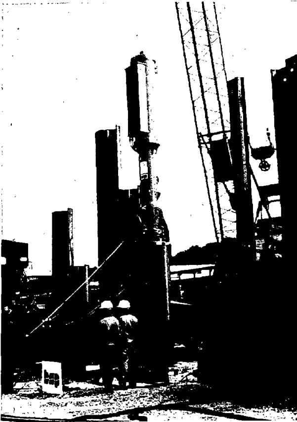
Fig. 5.1. -- BSP diesel hammer on sheet-wall piles.
