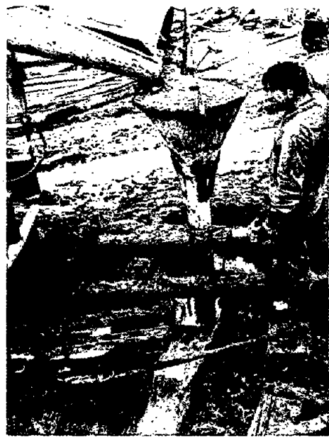
Fig. 16. -- Concreting with tremie.
