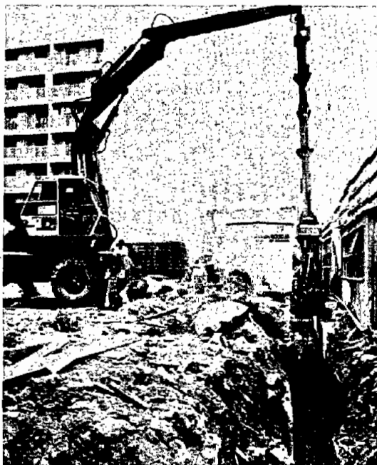
Fig. 10.13. -- Hydraulic bucket attached to end of extension arm.
