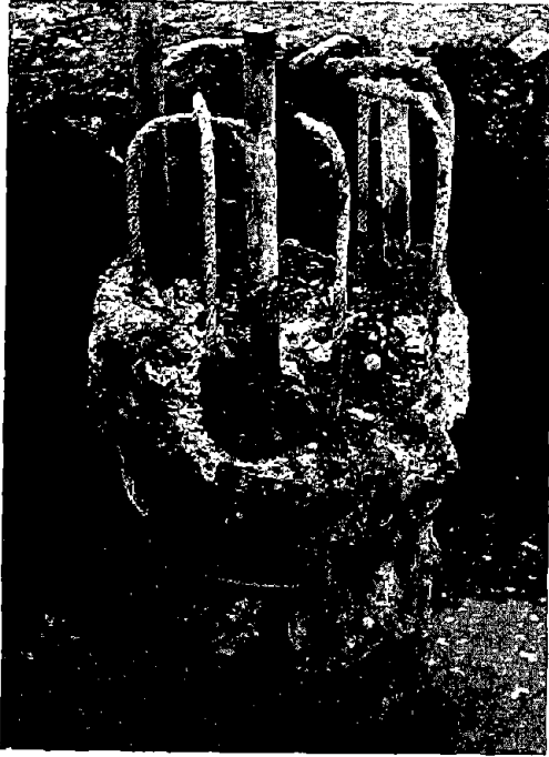
Fig. 181. -- Poor coating of reinforcing due to placement of insufficiently workable concrete.
