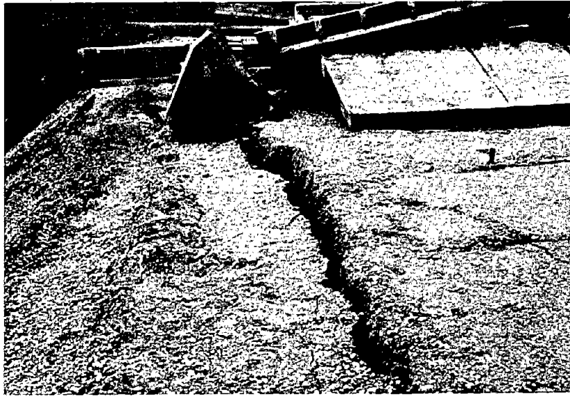
Fig. 41. -- Crack at the head of an embankment caused by construction of bored piles at the foot of embankment.
