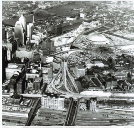
In 1964, the Crosstown Boulevard, a connector freeway skirting Pittsburgh, PA's, "Golden Triangle," was constructed using Federal-aid urban funding.
