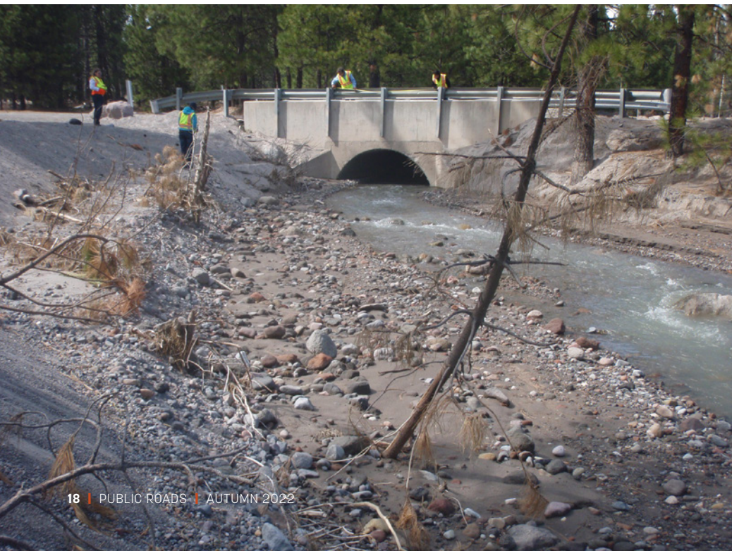
The upper section of the Mud Creek culvert shown in 2014 after extensive emergency removal of debris from a melting glacier on Mount Shasta in northern California. The initial debris removal partially restored creek flows until the entire structure was replaced with a bridge to withstand future events.
