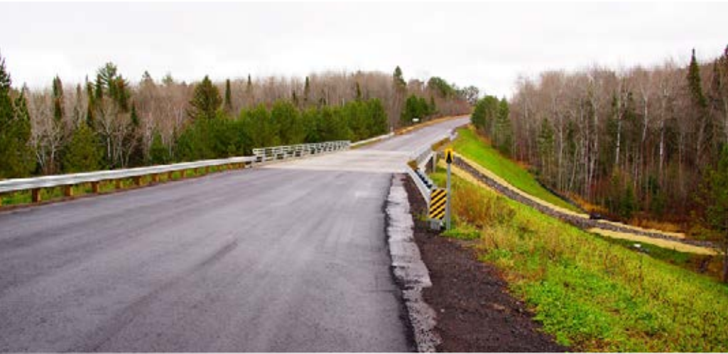
The ERFO Program funded a betterment project for the Fond du Lac Tribe in Minnesota, which included a new bridge rather than a replacement culvert. The bridge replacement option also has the secondary benefit of ensuring that fish passage would continue in the stream.
