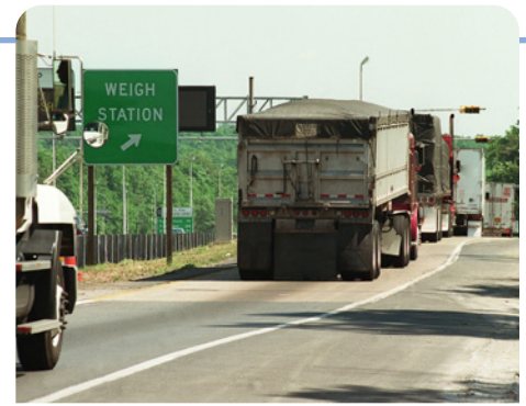
WIM technology uses in-road sensors or scales to help enforce commercial motor vehicle size and weight restrictions.
